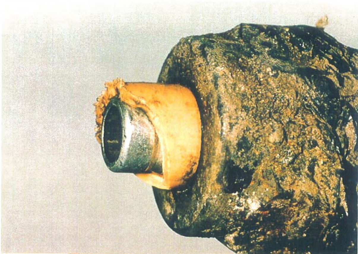
Figure 10 -- Close-up view of failed plastic pipe connection to steel tapping tee from site of Waterloo, Iowa, accident. A portion of the fractured plastic service line (light-colored material) remains attached to the tee.
