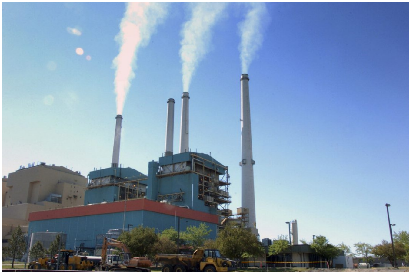
Smoke rises from the Colstrip Steam Electric Station, a coal burning power plant in
