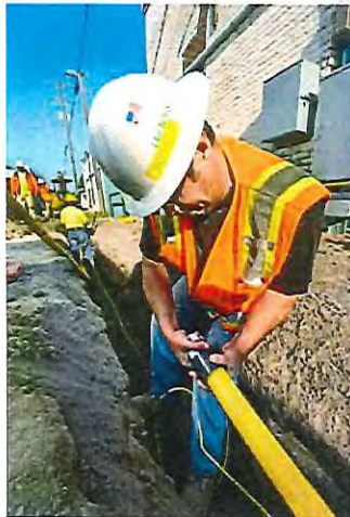
Aldyl A Natural Gas Pipe Replacement
