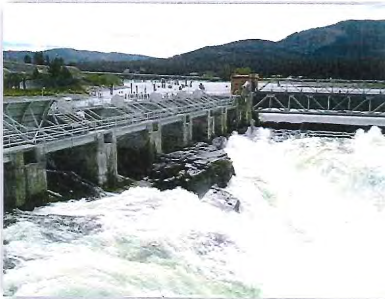
Post Falls Dam, Idaho
