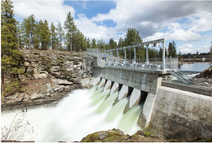
The 110-year old Post Falls South Channel Dam was officially returned to service after a two-year rehabilitation in February 2016.
