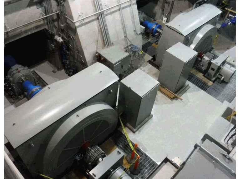
In 2016, the last two (of four) original turbine generating units at our 108-year-old Nine Mile Powerhouse were replaced with new, more efficient units as part of a multi-year project to increase the generation of clean, renewable, low-cost hydropower.
