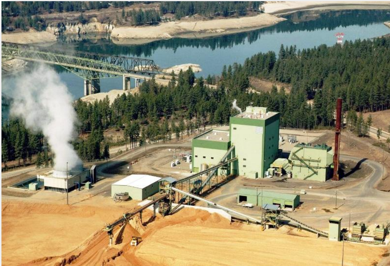
Kettle Falls Generating Station
