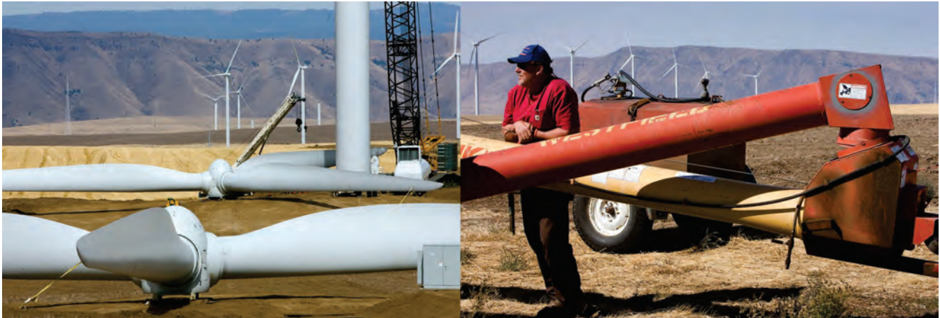
The first 76 Vestas turbines under construction at Biglow Canyon wind farm in 2007. Kevin McCullough, right, looked on enthusiastically at the time. He farms under about half of the wind farm's 217 turbines today and earns lease payments based on electricity production from the 13 turbines on land he and his wife own there. (File photos by Ross William Hamilton)
