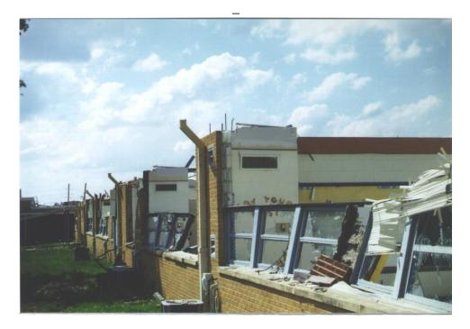
ES: DOD 8: Uplift of entire roof structure and collapse of non-bearing walls
