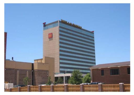
MRB: Generally rectangular shapes; flat roof with parapet and penthouse; BUR or single-ply membrane with or without gravel; metal deck, poured gypsum or concrete deck; glass or metal curtain walls, marble panels or pre-cast concrete wall panels
