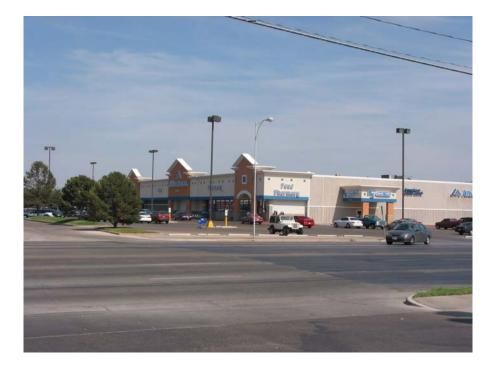
LIRB: Flat roof with built-up tar and gravel roofing; 2-3 ft parapet; metal roof deck with rigid insulation; light steel roof structure; tilt-up concrete panel walls; glass store front
