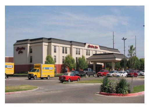
M: Less than five stories; one or more rectangular modules; flat, gable, hip or mansard roof; asphalt shingles, tile, slate or BUR covering; plywood or metal roof decking; stud walls with EIFS, stucco or wood siding or brick veneer; canopy over driveway at entrance; exterior walkways or balconies
