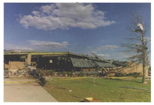
ES: DOD 9: Collapse of load-bearing walls
