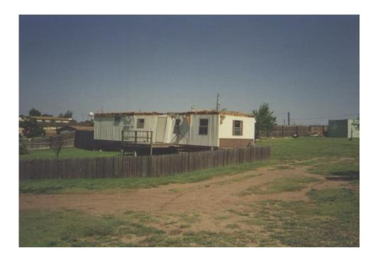
MHSW: DOD 4: Complete uplift of roof; most walls remain standing
