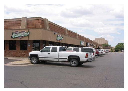
SM: Long, rectangular, single-story building; flat roof with parapet; BUR or single-ply membrane roof system with rigid insulation; wood, metal or wood-fiber cement roof panels; concrete block walls or stud walls with brick veneer; large glass windows and glass entry doors; canopy or covered walkway attached to building
