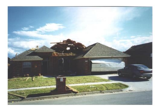
FR12: DOD 4: Uplift of roof deck and loss of roof covering (>20%); garage door collapses outward
