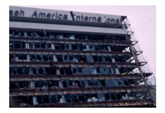
MRB: DOD 9: Significant damage to curtain walls and some interior walls
