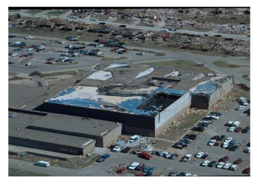
LSM: DOD 4: Uplift of some roof decking; significant loss of roofing material (>20%); loss of rooftop HVAC
