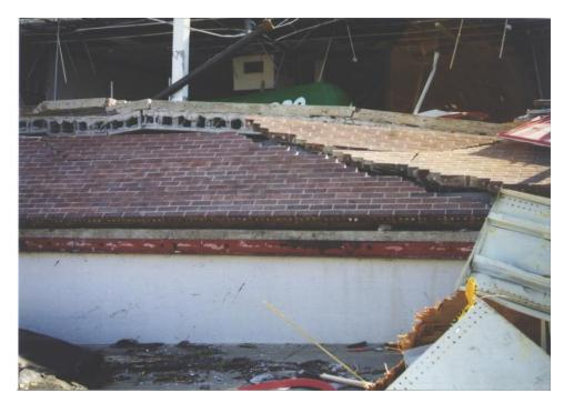
WHB: DOD 5: Collapse of non-bearing exterior wall
