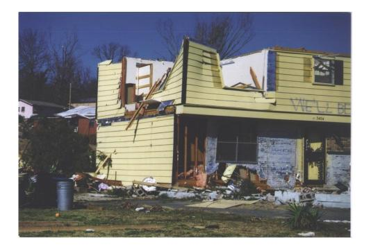
ACT: DOD 4: Uplift or collapse of roof structure leaving most walls standing
