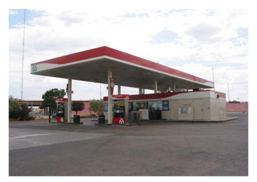
SSC: Large rectangular free-standing canopy supported on columns; metal panels cover bottom side of canopy; metal or plastic fascia materials cover perimeter of canopy
