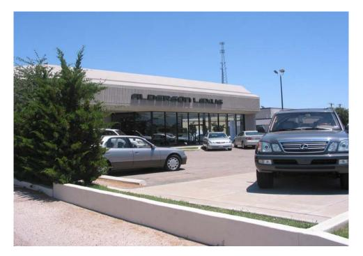
ASR: Single story with flat roof; BUR or single-ply membrane; metal or plywood roof deck; stud walls with EIFS, stucco or tilt-up panels
