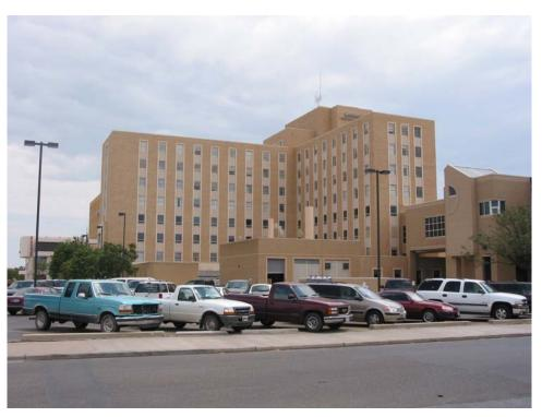
IB: Height from 1 to 10 stories; single-ply membrane, polyurethane foam or metal roof systems; masonry, cut-stone or pre-cast wall panels; balconies, porches or porticos; heavy façade; relatively small windows
