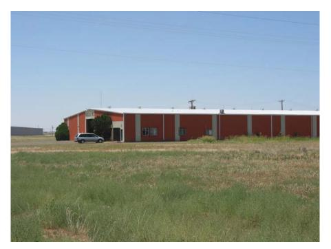
MBS: Metal roof and wall panels; gable roof shape; Z or C-shaped purlins and girts; single-bay rigid frames; x-bracing parallel to ridge
