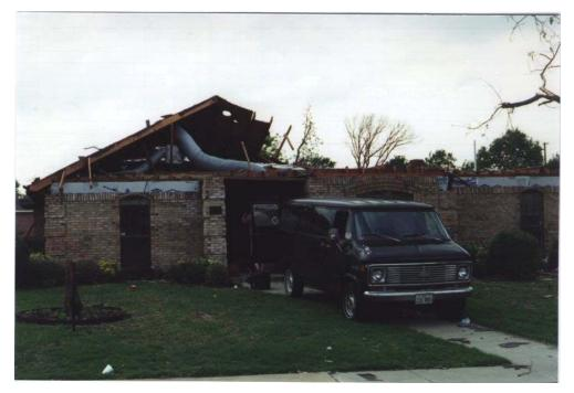
FR12: DOD 6: Large sections of roof removed; most walls remain standing
