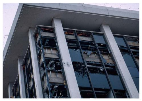
MRB: DOD 5: Broken glass in curtain walls; damage to building interior
