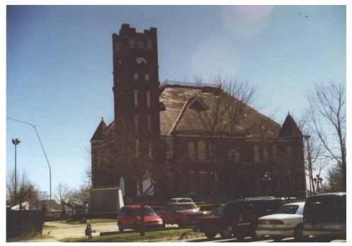
IB: DOD 5: Uplift of light-weight roof deck and insulation; significant loss of roofing material (>20%)
