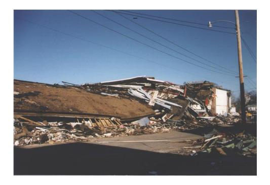
LIRB: DOD 6: Long span roof structure collapses downward
