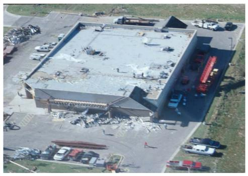
LIRB: DOD 2: Significant loss of roofing material; loss of rooftop HVAC
