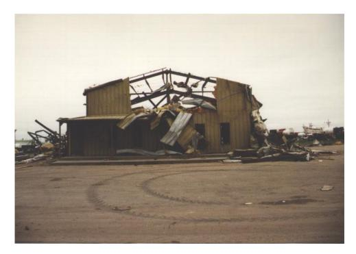
MBS: DOD 7: Progressive collapse of rigid frames
