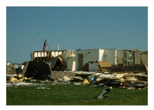
FR12: DOD 7: Top floor (First floor in this case) exterior walls collapsed
