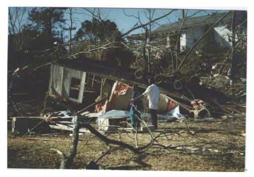
MHSW: DOD 9: Complete destruction of unit; debris blown away
