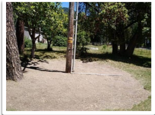
Figure 36: Pole Clearing at Pole Base
