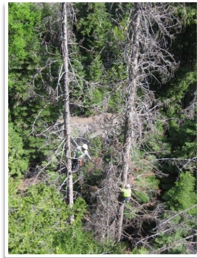
Figure 32: Hazard Tree Removal
