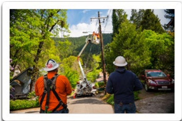
Figure 60: Line Workers Performing Work
