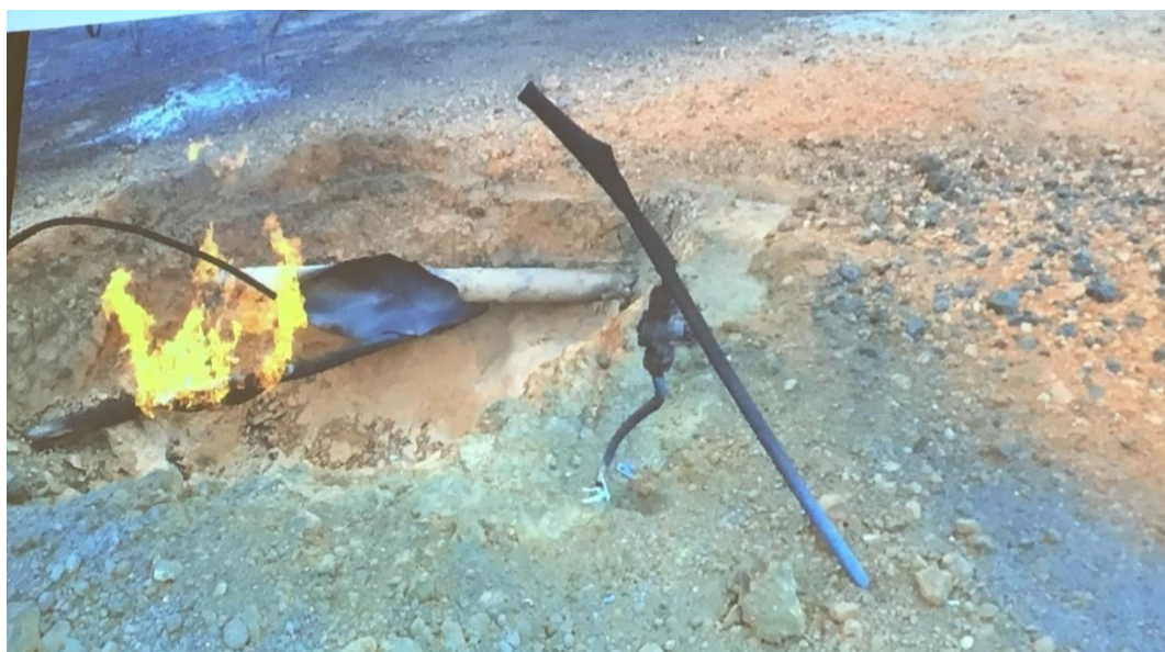
Figure 1: Small Diameter Gathering and Gas Transmission Pipeline
