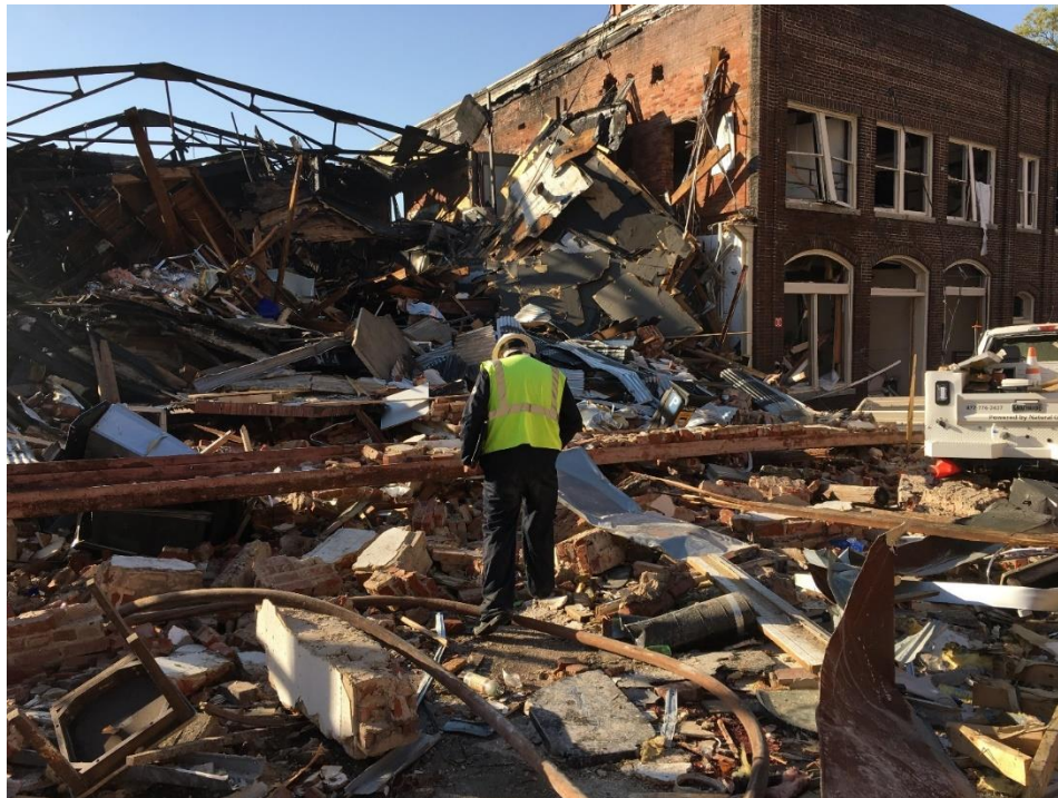
Figure 4: Durham, NC Gas Explosion
