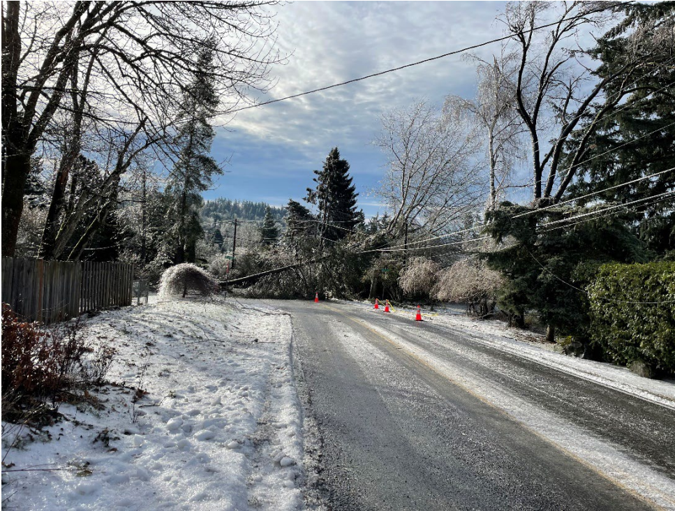
Figure 1: Photo of Uprooted Tree, Damaged Electric Lines, and Icy Road
