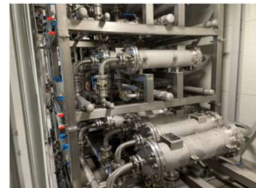
Membranes to clean RNG at Tyson Lexington facility (NW Natural project)
