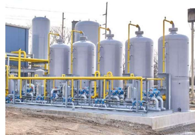
Nitrogen removal system for large landfill RNG project
