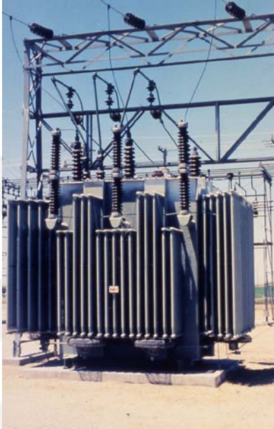
Substation transformer with load tap changer
