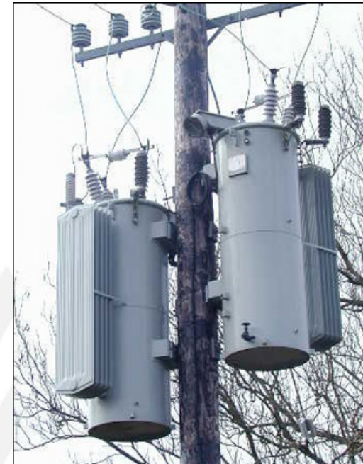
2 Single Phase Voltage Regulators
