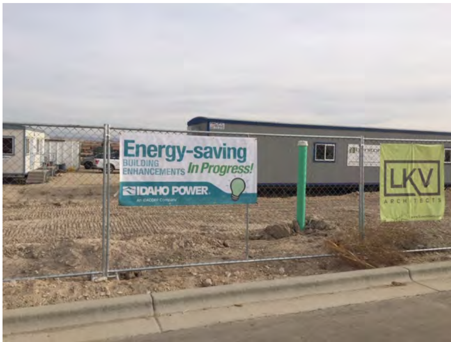
Figure 26. Energy-efficiency banner display at Kuna School District building site
