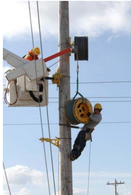
Idaho Power linemen install upgrades.
