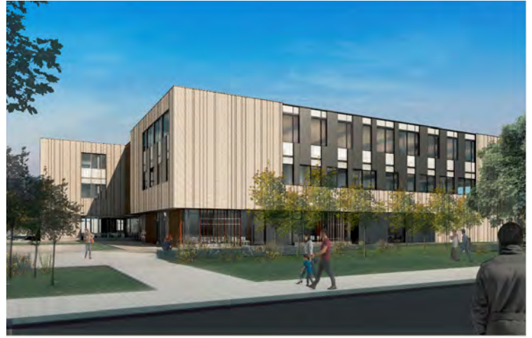
view from the north - daytime
