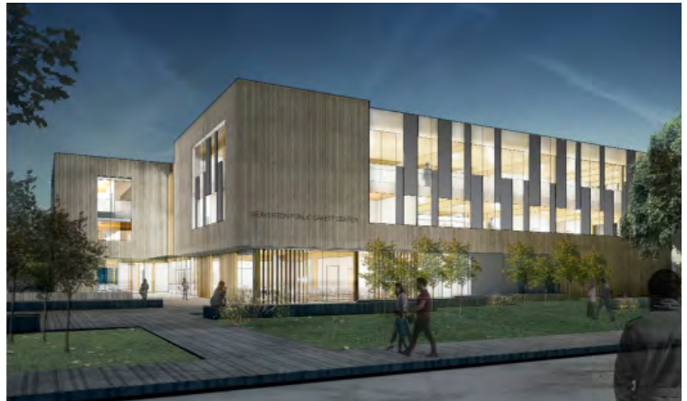
view from the north - nighttime
