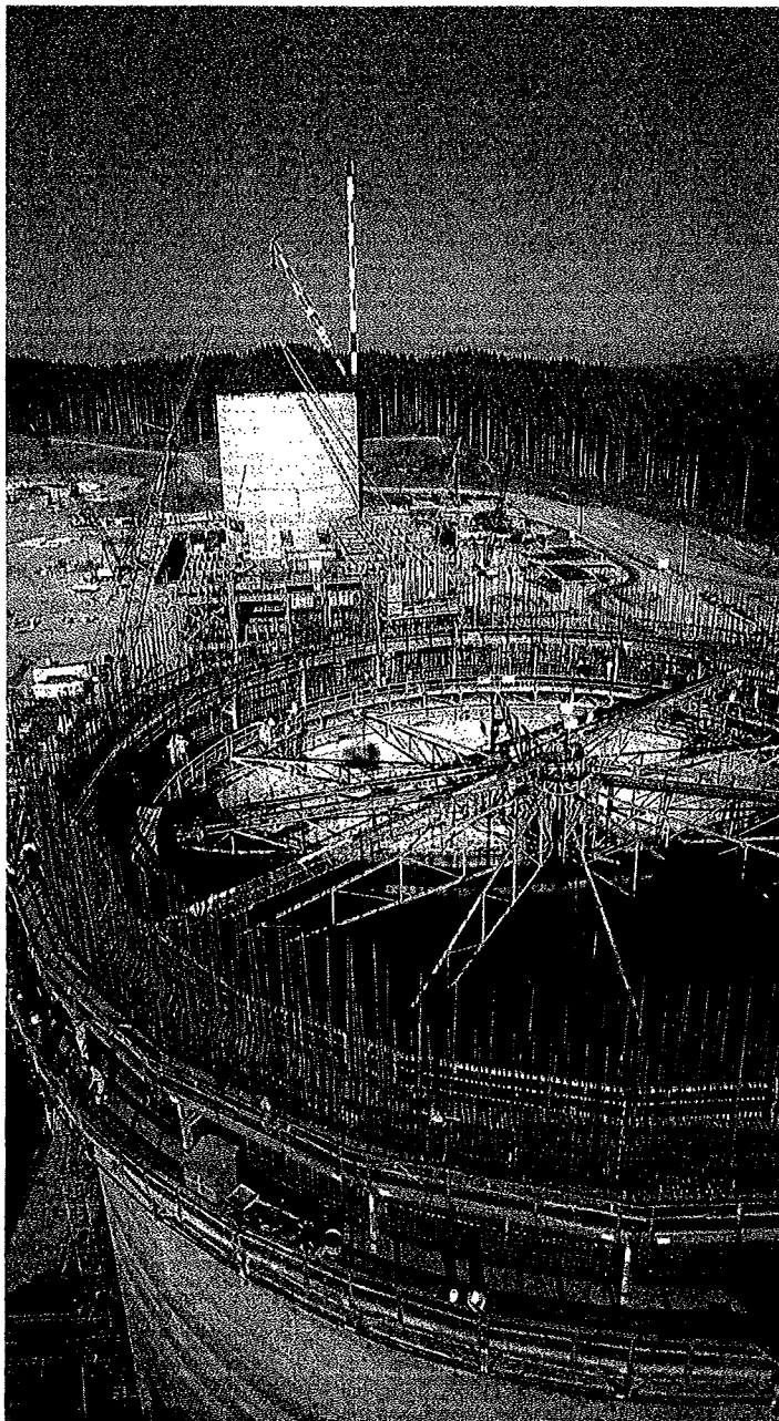
PGE is a 10 percent partner in the Washington Public Power Supply System's 1240-megawatt nuclear plant being built near Montesano, Washington.
