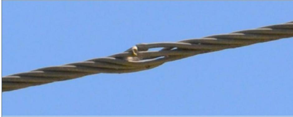
**Figure 29. Damaged Conductor Identified by EFD System**
