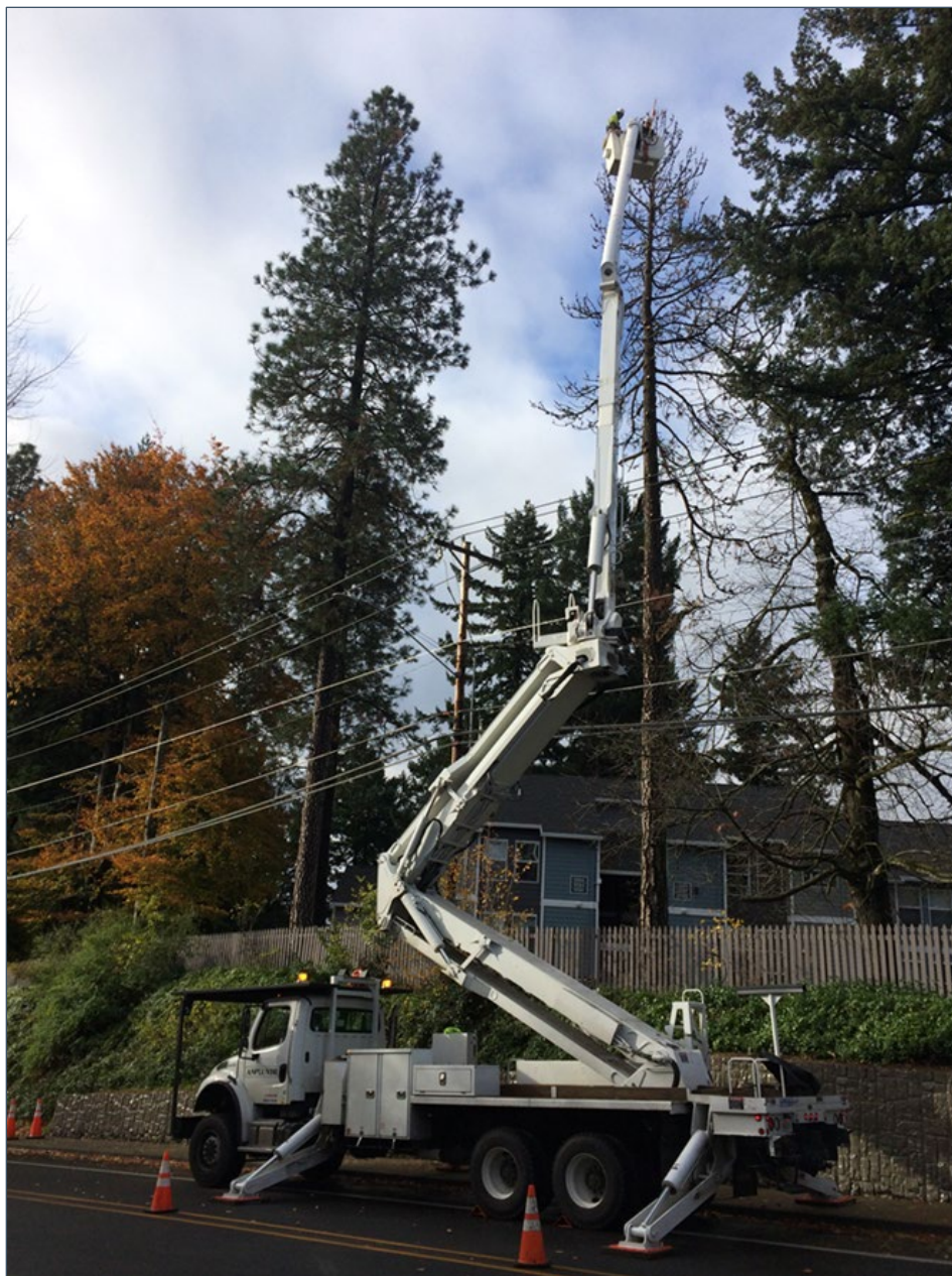
Figure 24. Aerial Lift Removing Dead Tree on Border of AWRR Zone
