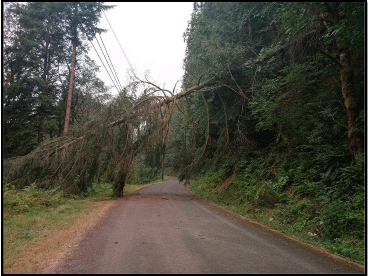
Figure 17: Fallen Tree Across Power Line
