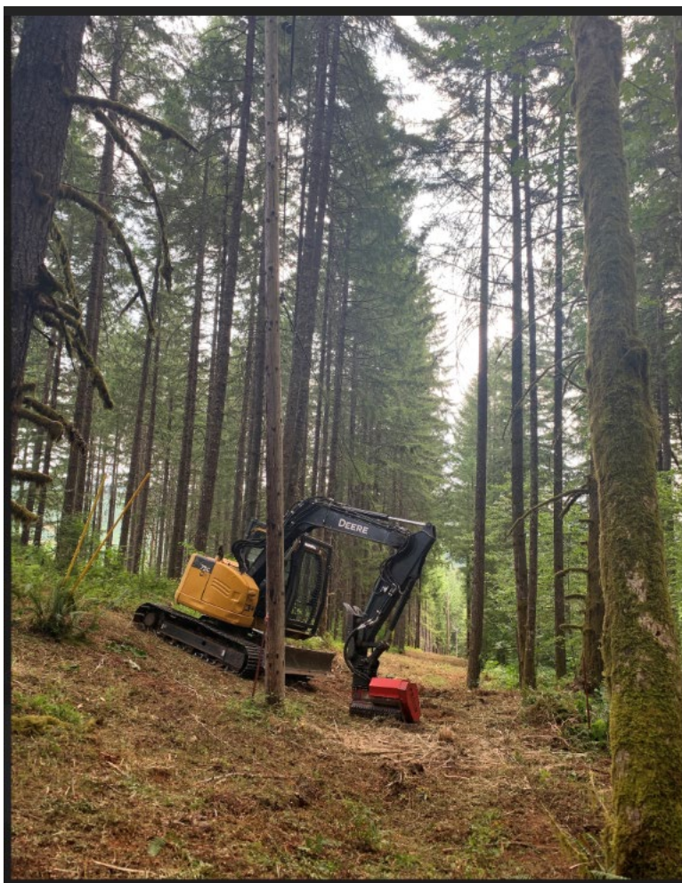
Figure 16: SlashBuster Clearing Right-of-Way
