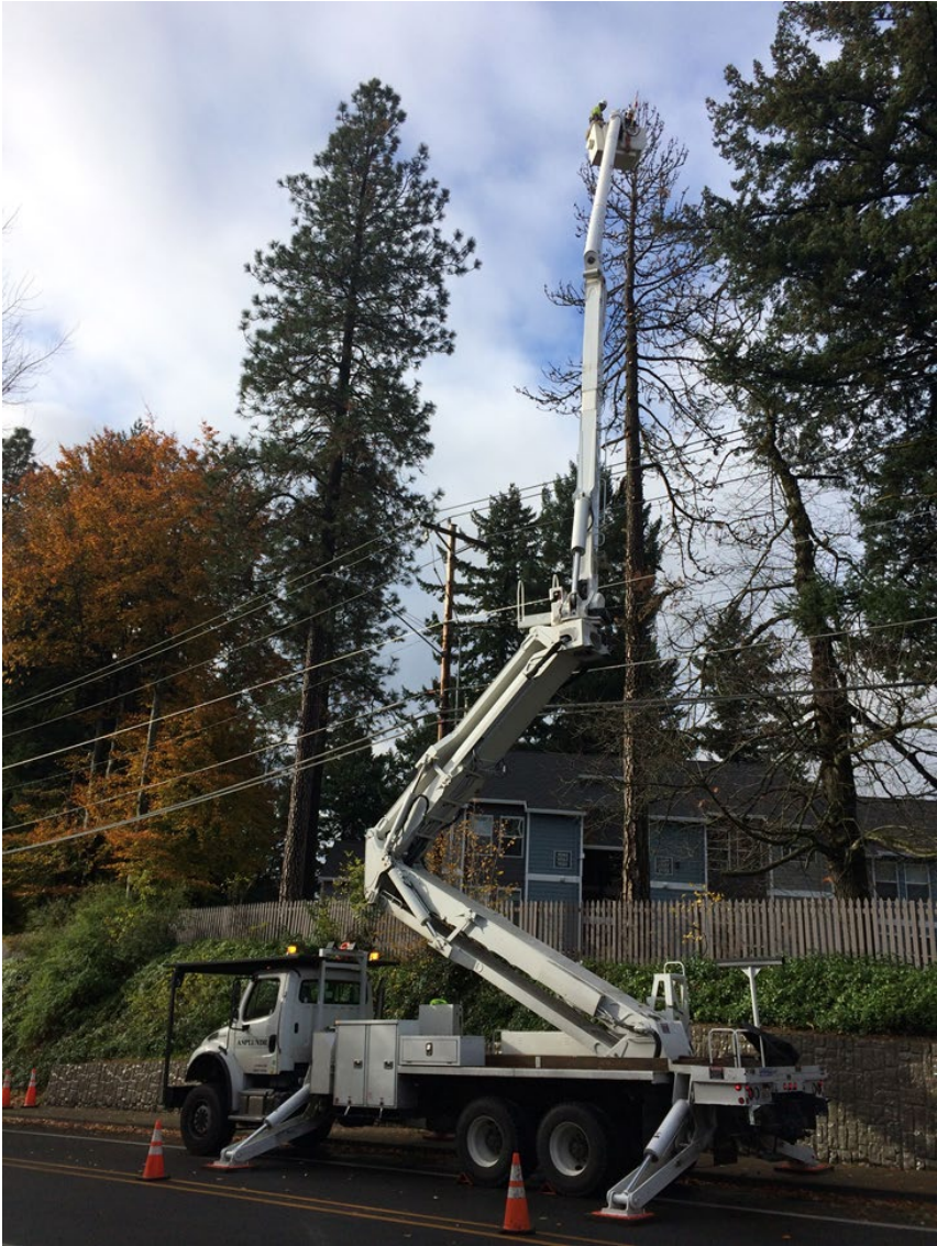
Figure 17: 105' Aerial Lift Removing Dead Tree on Border of AWRR Zone
