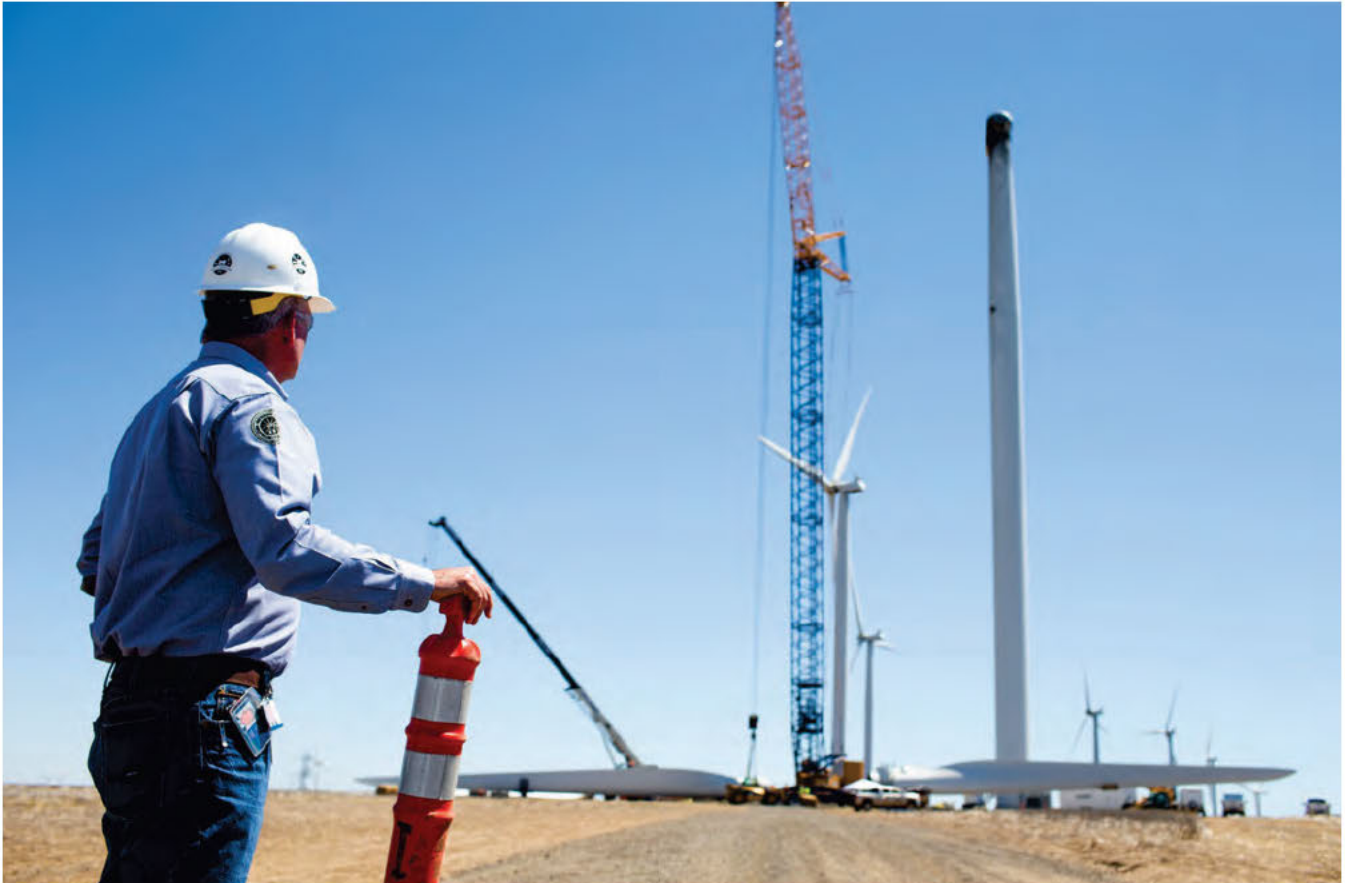
Brad Jenkins, PGE's vice president of utility operations, watches as workers install new blades in late June on the Vestas turbine that threw a blade on Feb 1.
