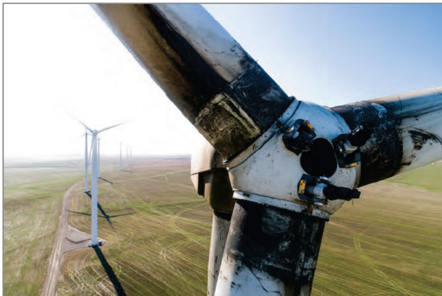
A metal frame and pieces of fiberglass fell from the spinner cone of this Vestas turbine into a field below at Biglow Canyon wind farm in April 2021. PGE didn't report the incident to regulators until this summer. Wind
