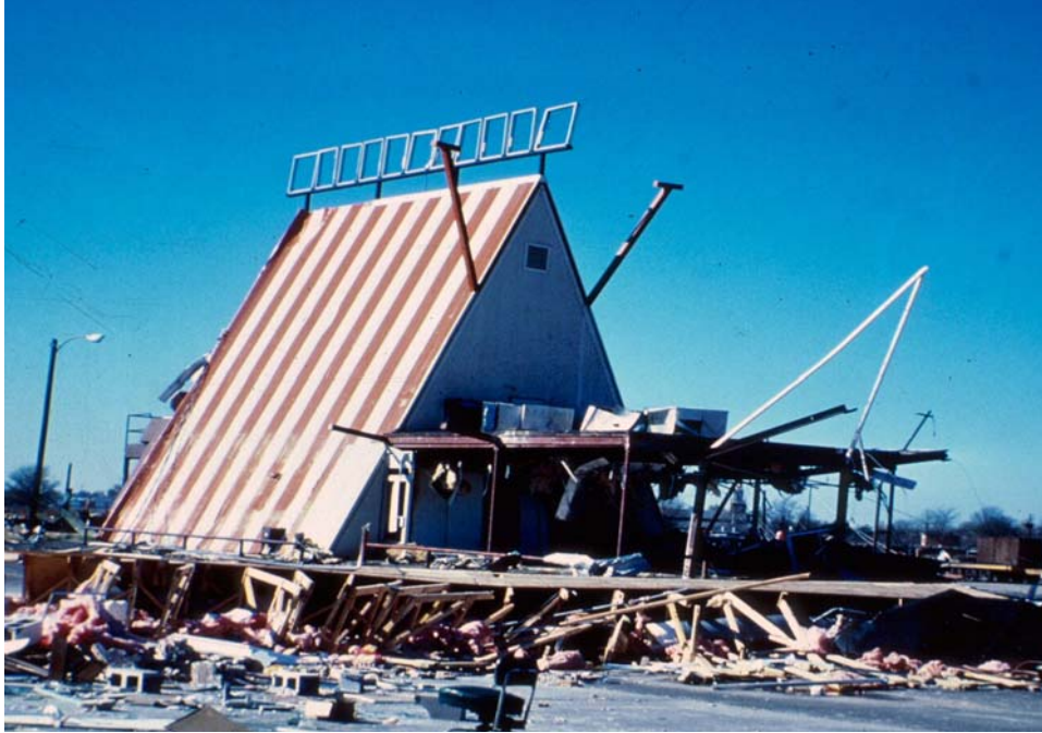
SRB: DOD 5: Canopies and covered walkways destroyed
