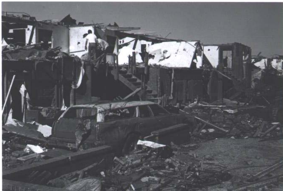
ACT: DOD 5: Most top story walls collapsed
