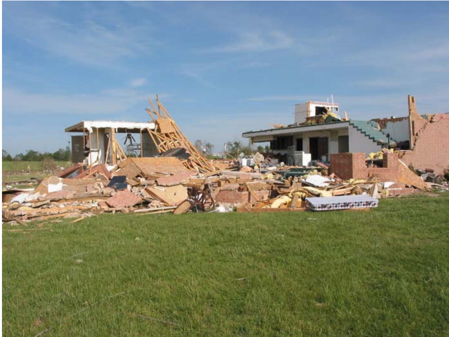
FR12: DOD 10: Total destruction of entire building
