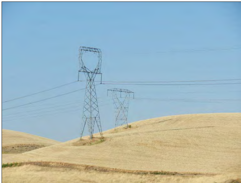
Figure 5-4. Photograph Showing a Harvested Wheat Field with existing Transmission Line Structures Present within the Field. Towers located on hillsides may result in less farmable acreage compared to placement on flat ground because of reduced equipment maneuverability.
