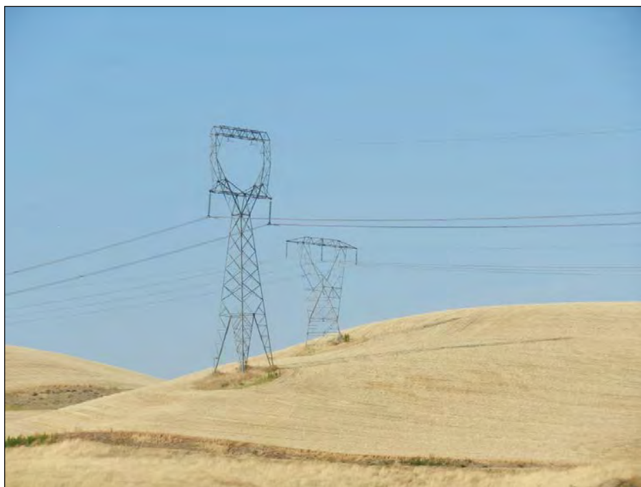
Figure 5-4. Photograph Showing a Harvested Wheat Field with existing Transmission Line Structures Present within the Field. Towers located on hillsides may result in less farmable acreage compared to placement on flat ground because of reduced equipment maneuverability.
