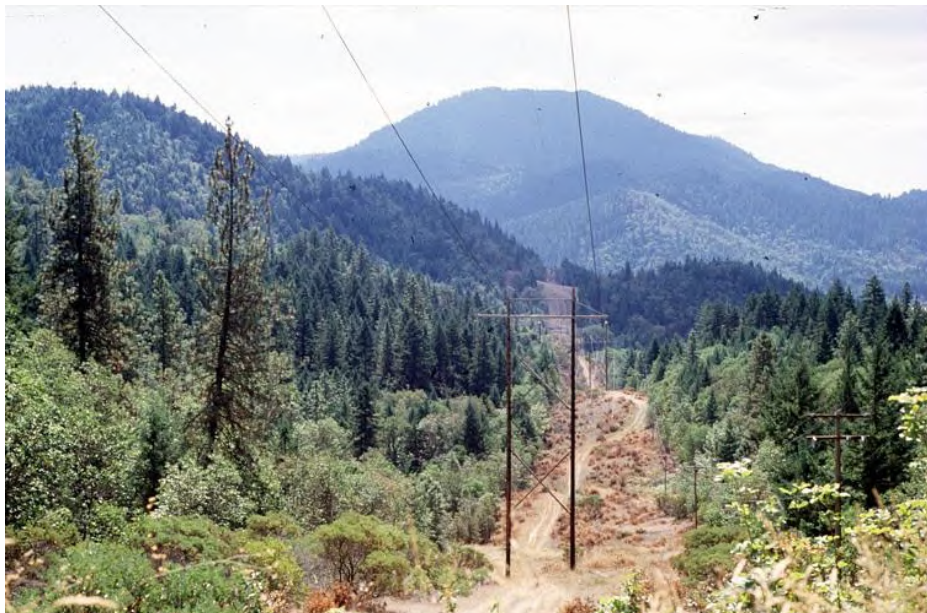
Figure 7.2. Incompatible species treated in the Line 72 right-of-way in, Oregon two years after reclamation. Herbicide treatments help maintain the right-of-way and are used to convert it to a wire zone-border zone prescription (Figure 6.3)
