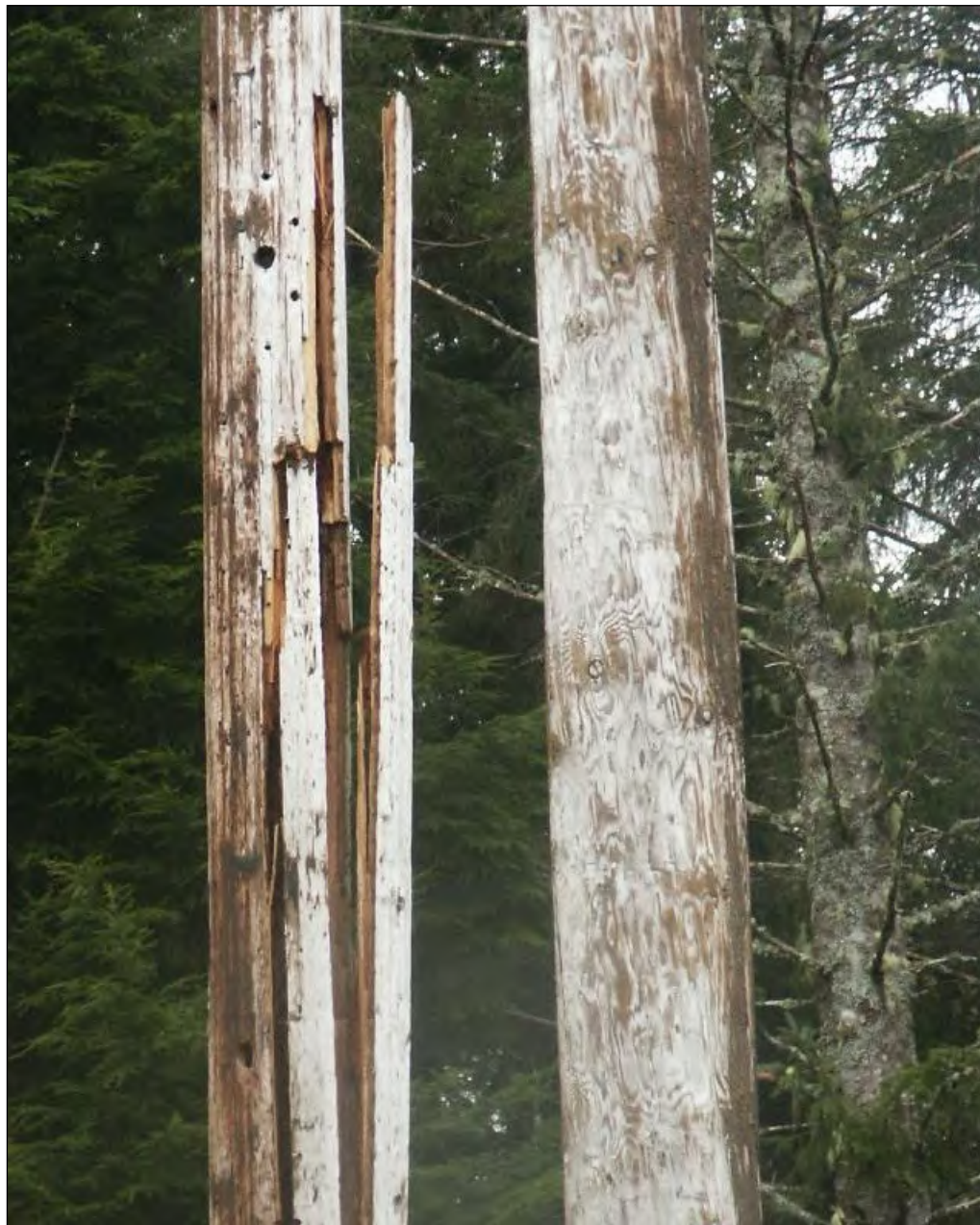
Figure 2.6. Cracked pole – an example of the type of conditions tree crews should report.
