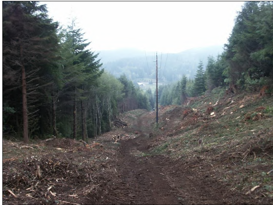
Figure 6.2. Line 4 in California following work (note the trees mid-span where the line is more than 100-feet off the ground).
