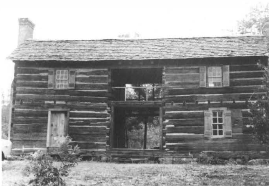
Looney House, Asheville vicinity, St. Clair County, Alabama. Examples of vernacular styles of architecture can qualify under Criterion C. Built ca. 1818, the Looney House is significant as possibly the State's oldest extant two-story dogtrot type of dwelling. The defining open center passage of the dogtrot was a regional building response to the southern climate. (Photo by Carolyn Scott).
