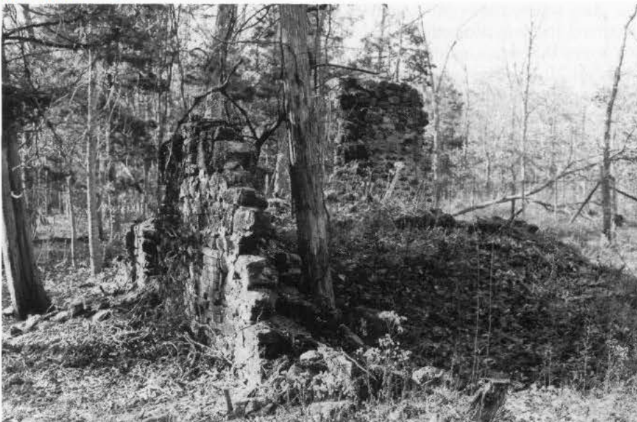
Figure 21: The Melting Furnace Site, part of the Estellville Glassworks Historic District, is in Atlantic County, New Jersey. Cemented with limestone mortar, it was constructed of sandstone and aggregated stone. All four walls of this structure were once pierced with large arched openings in brick. The site displays integrity of workmanship because of its standing wall surface, showing the brick arched colonnade. (Karen DeRosa)
