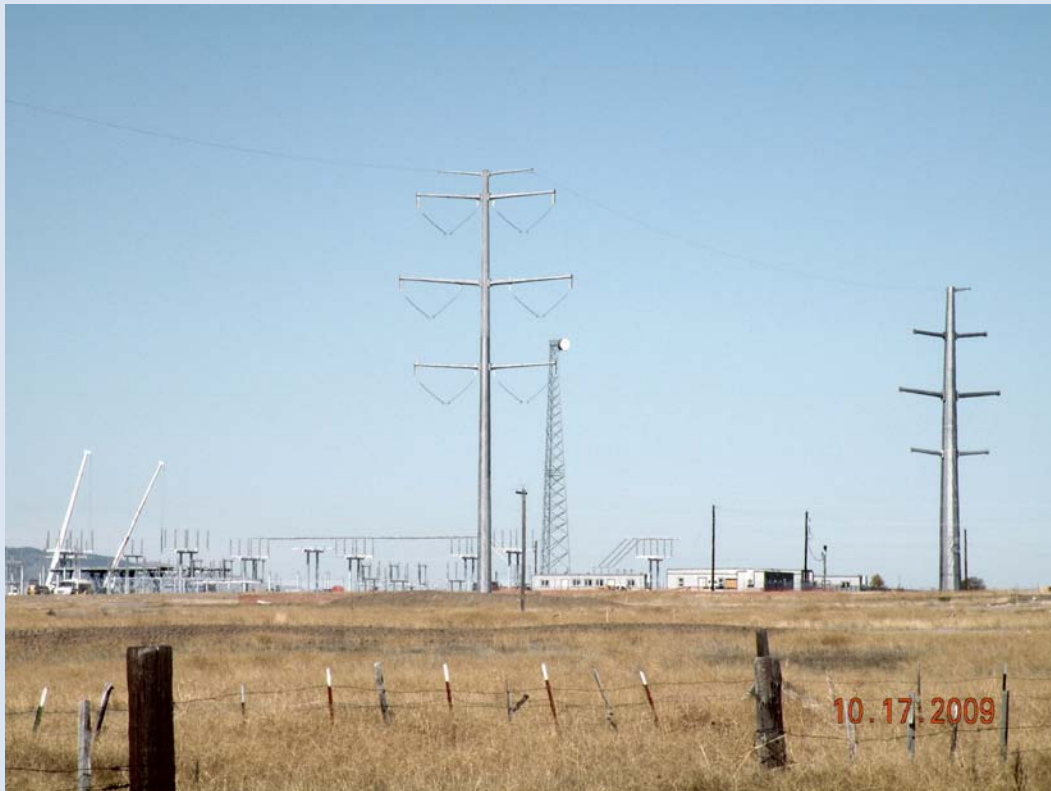
Gateway Central Project under Construction at the Populus Substation in Idaho
