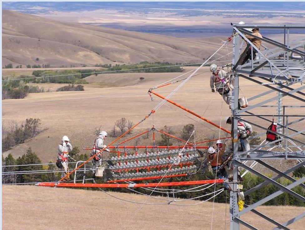
High-Voltage Transmission Construction in Montana
