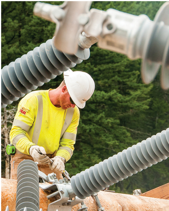
Journeyman lineman prepares equipment for upgrade of NorthWestern Energy's Jack Rabbit-Big Sky Project. Photo courtesy of Susan Malee, NorthWestern Energy
