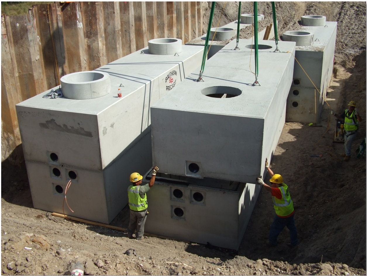
Figure 3: Typical Splicing Vault Installation (lower voltage example)
