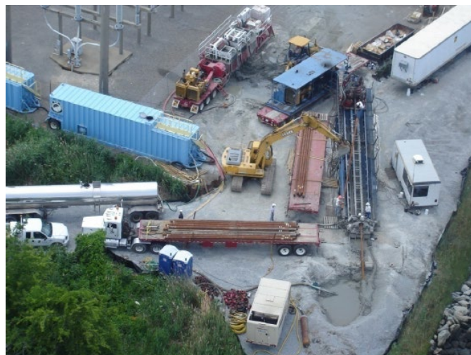
Figure 8: Typical HDD Setup (Lower Voltage Example)
