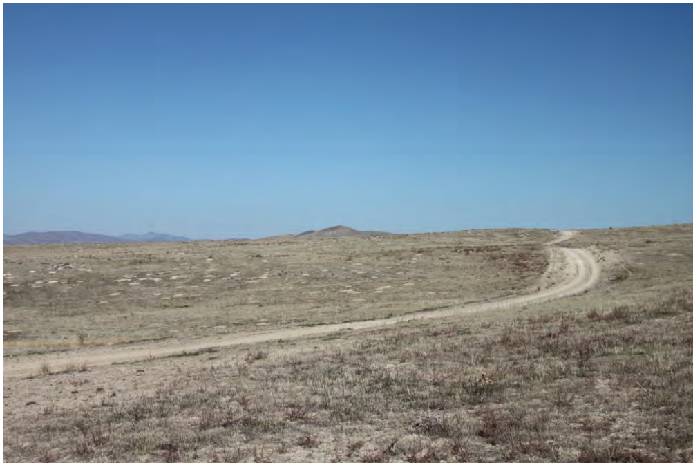
IOP 4-6 (Graded gravel road, looking northwest)
