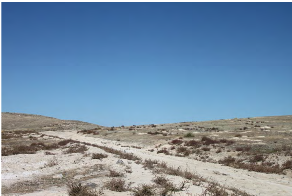
IOP 4-7 (Graded gravel road, looking north)
