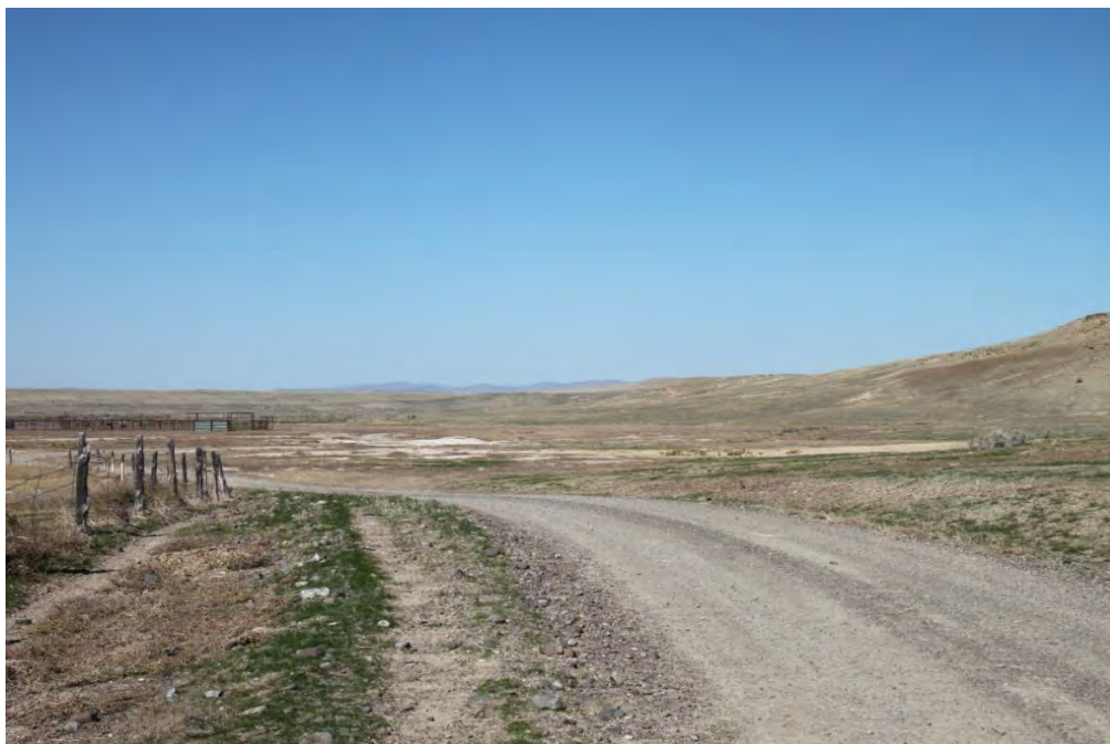
IOP 4-8 (Graded gravel road, looking north)
