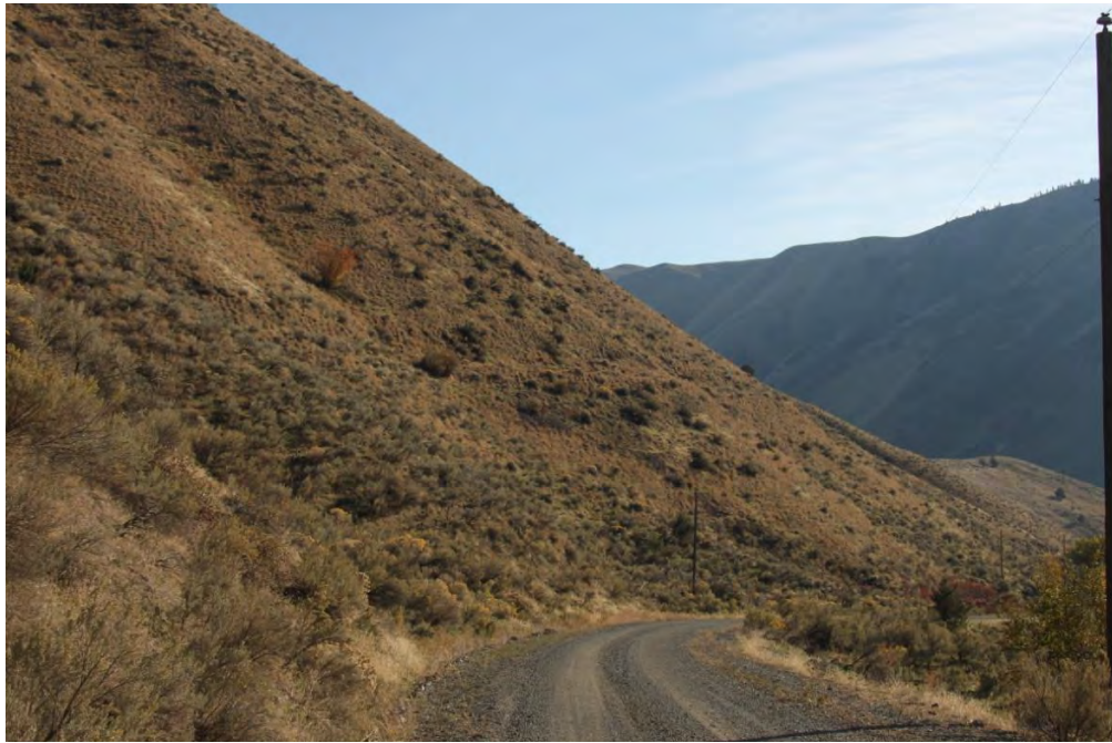
IOP 3-10 (Plano Road, single pole transmission line, looking southwest)
