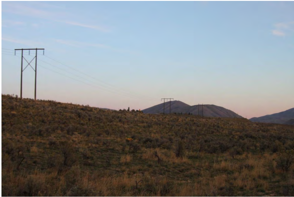
IOP 3-7 (H-Frame transmission line, looking southeast)
