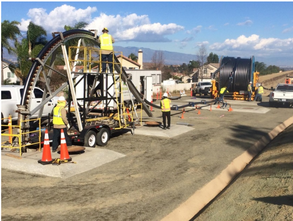
Figure 4: Typical Cable Pulling Setup
