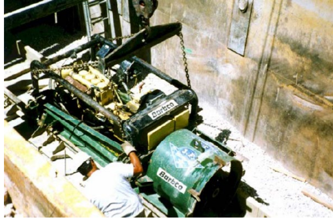
Figure 7: Typical J&B Setup (Lower Voltage Example)
