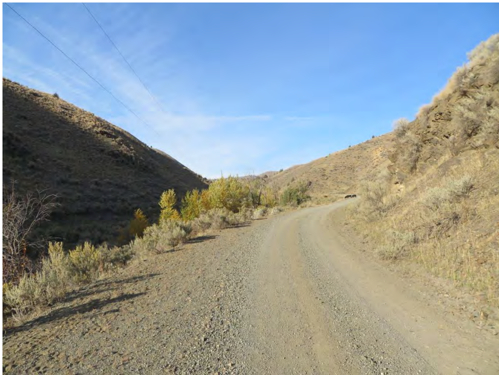
IOP 3-10 (Plano Road adjacent to Sisley Creek, looking north)
