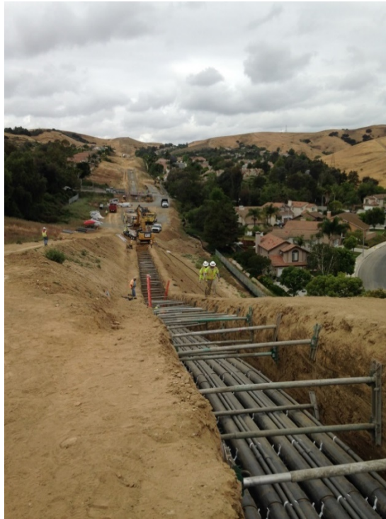
Figure 5: Typical Trench Excavation (Single Trench Only)
