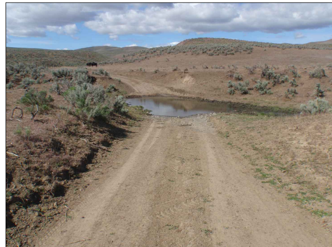
SITE PHOTO - FACING NORTH (MAY '14)
