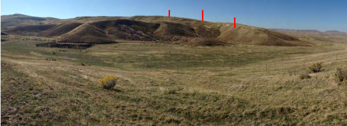
Photo 2: Looking south into the toe of landslide complex; approximate locations of towers 204/2 through 204/4 shown for reference.
