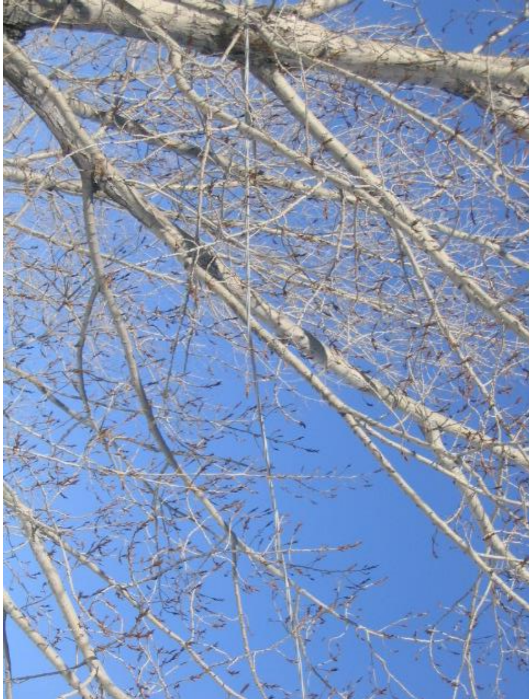
Figure 5.1. Trees with branches applying sufficient pressure to cause damage to insulated service and street light lines should be pruned on cycle to relieve the pressure.
