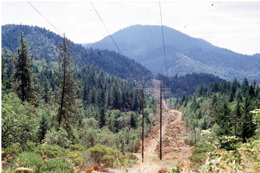
Figure 7.2. Incompatible species treated in the Line 72 right-of-way in, Oregon two years after reclamation. Herbicide treatments help maintain the right-of-way and are used to convert it to a wire zone-border zone prescription (Figure 6.3)
