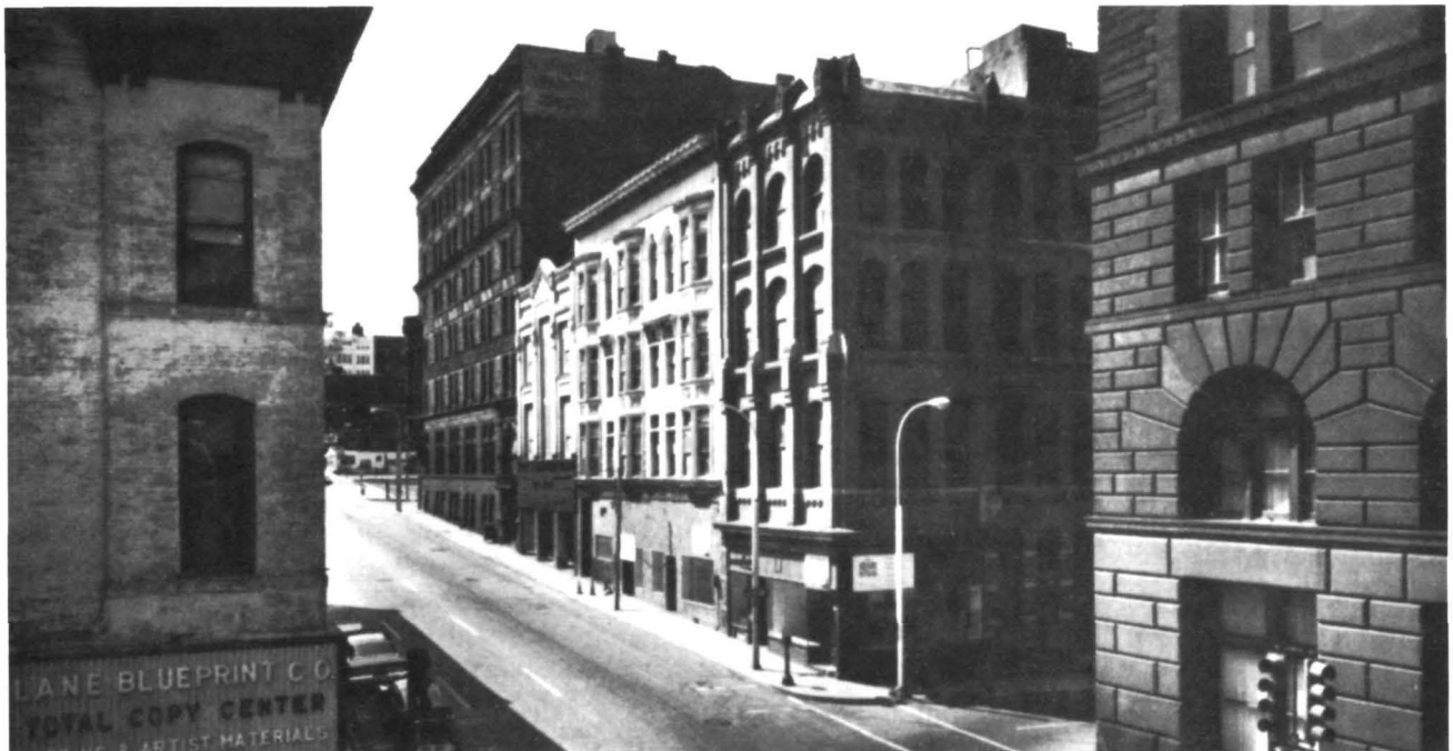
Older commercial buildings in downtown areas are particularly vulnerable to decay and demolition yet could be successfully rehabilitated. This downtown block, in Kansas City, Missouri, is listed in the National Register of Historic Places as part of the West Ninth Street/Baltimore Avenue Historic District. (Paul S. Kivett)
