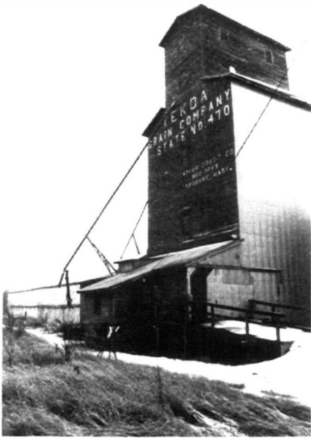
The Tekoa Grain Company Elevator and Flat-house, Whitman County, Washington, is one of several properties listed in the National Register as part of the multiple property group, Grain Production in Eastern Washington. (Holstine)
