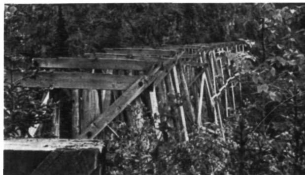
Engineering structures associated with transportation lines, whether currently used or not, should be included in the survey. The Copper River and Northwestern Railway, Chitina vicinity, Alaska, was constructed to gain access to the interior copper country and thus, is closely associated with a major economic activity in this area. The National Register of Historic Places listing includes 25 miles of railroad bed, sections of track, trestles, and associated buildings. (Alaska Division of Parks)
