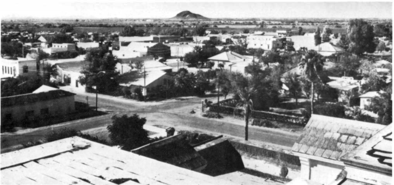
The certification of local governments under the National Historic Preservation Act has made it possible for historic preservation programs operated by local governments, as in Florence, Arizona, to exercise greater autonomy in nominating properties to the National Register of Historic Places and in other preservation activities, such as survey and inventory, and comprehensive planning. (Harris Sobin)
