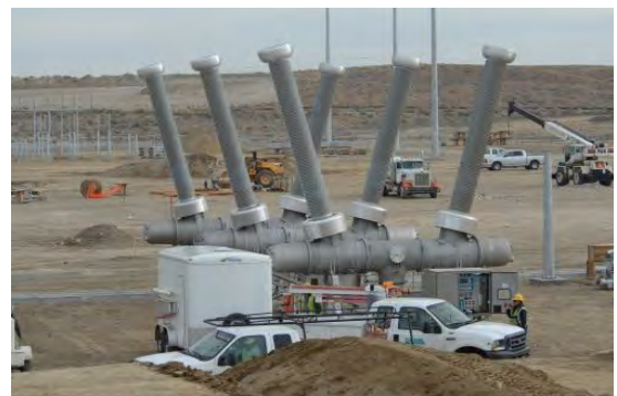
Transmission lines under construction at the Hemingway substation.
