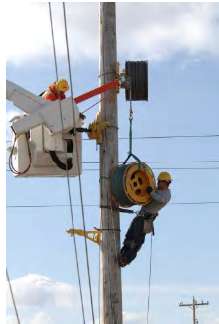
Idaho Power linemen install upgrades.
