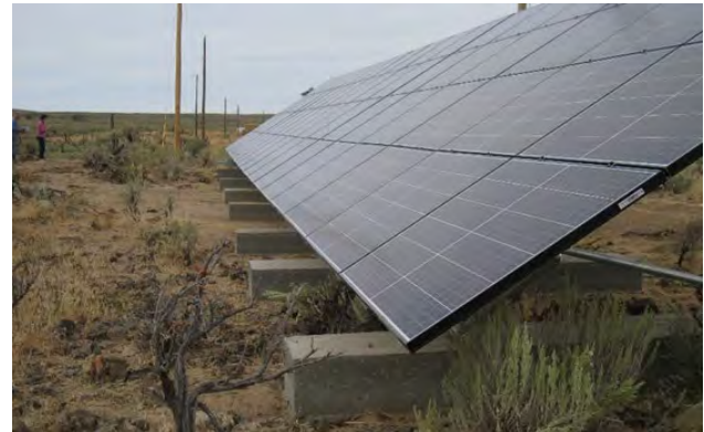
Solar installation as part of the Solar End-of-Feeder Pilot Project.
