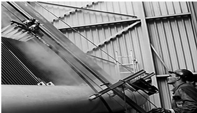
Fig. 3 Semi-Automated pressure cleaning.
