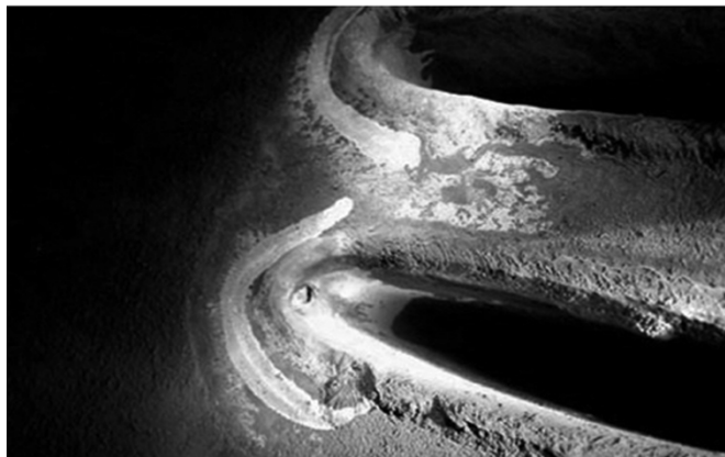
Fig. 2 DHACI Indices 1-5 for upper ducts and tube entries.
