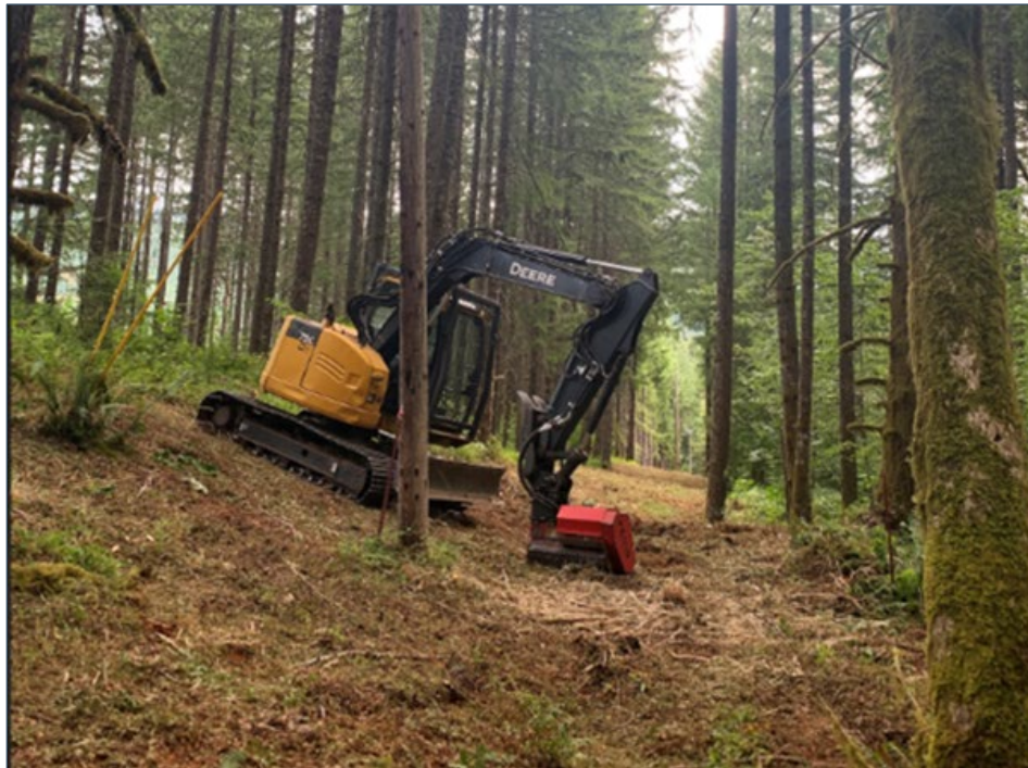
Figure 23. SlashBuster Clearing Right of Way
