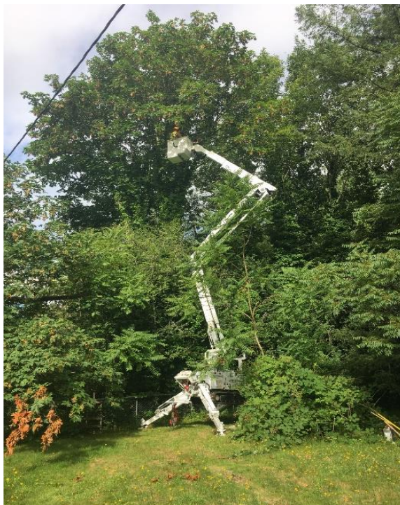
FIGURE 11: FORESTRY BUCKET AND TREE-TRIMMING CREW ON AWRR DEPLOYMEN
