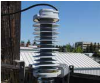
Siemens Type 3EK distribution class surge arresters with an Arc Protection System (APS)
