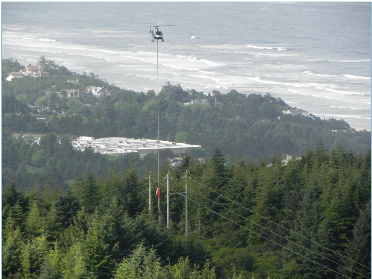
Aerial trimming of Central Lincoln’s transmission right-of-way
