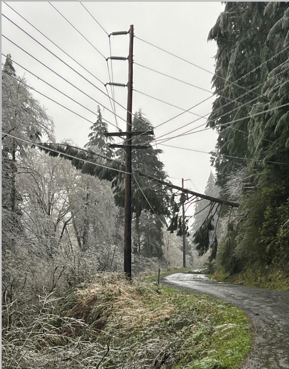
Tree from outside the right-of-way in the lines
