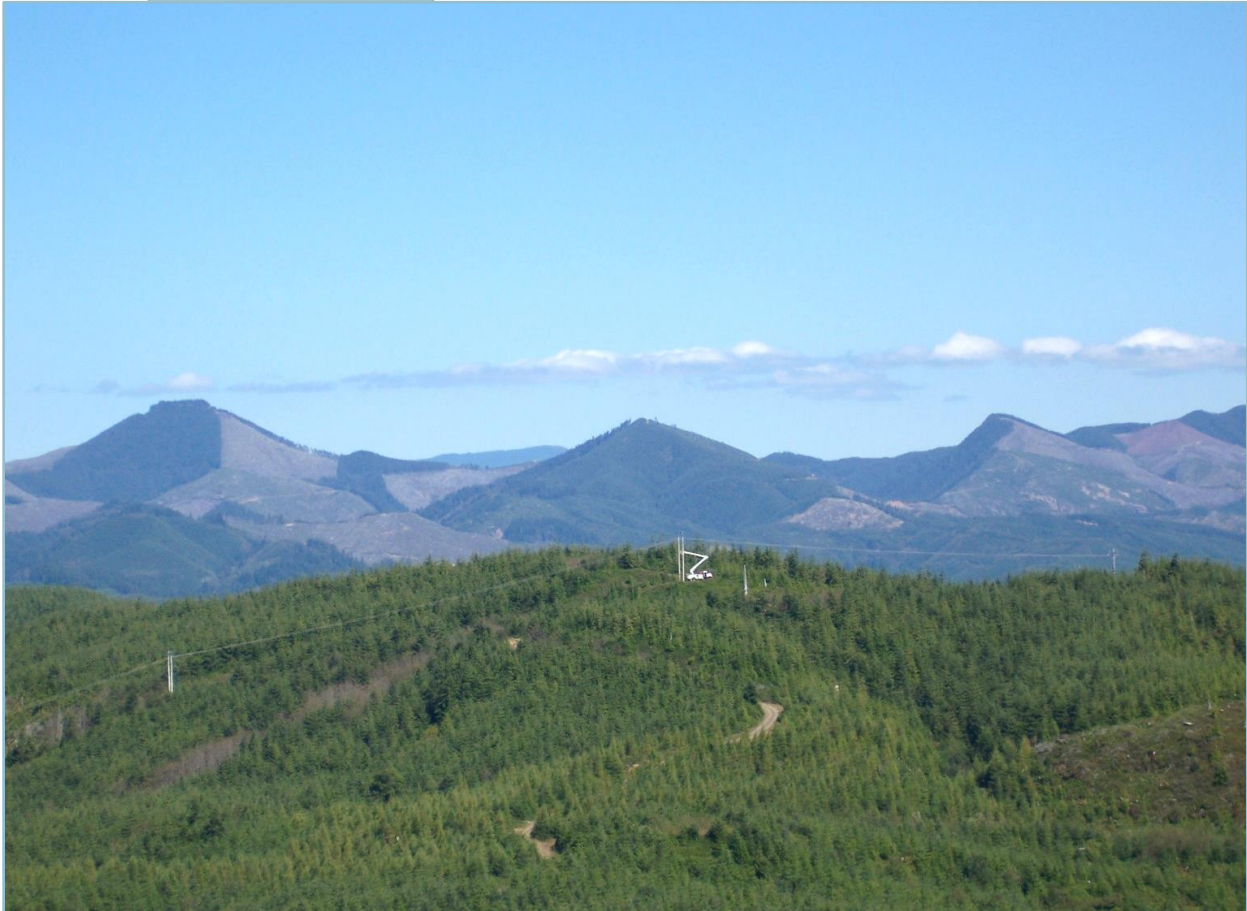
Transmission line serving the northern portion of Central Lincoln's service area
