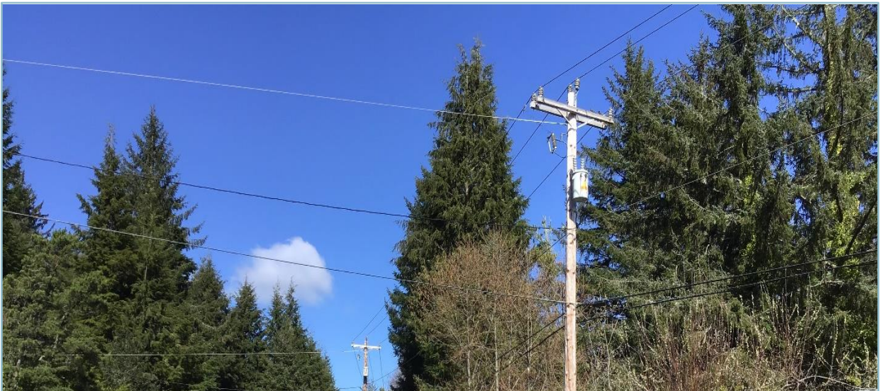
Distribution lines in Central Lincoln service area
