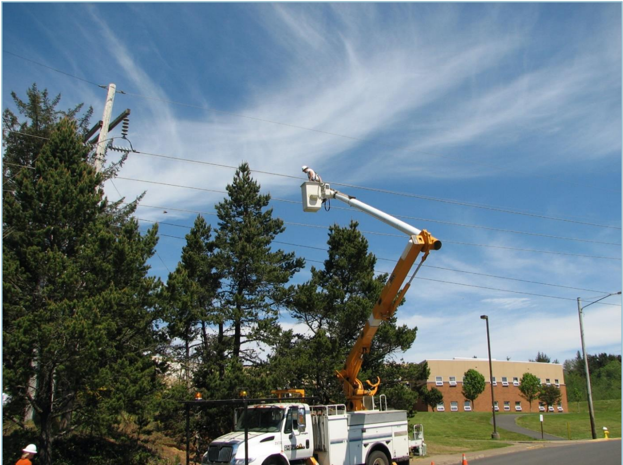
Central Lincoln tree crews
