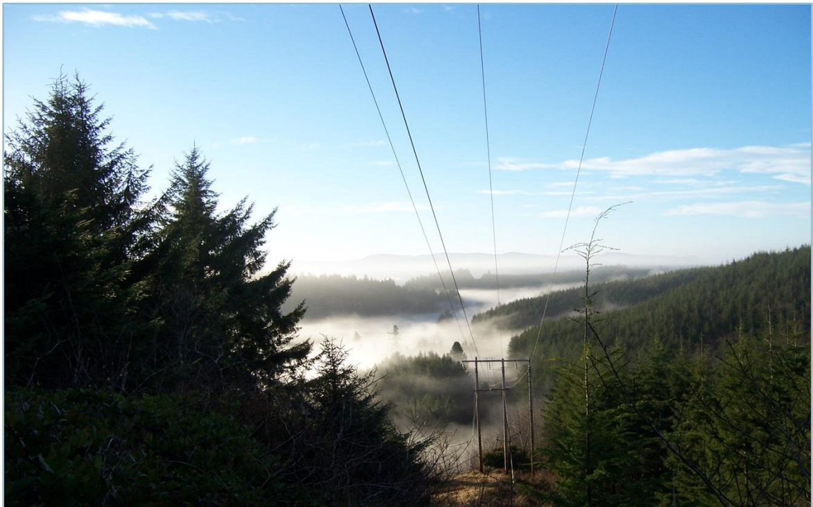
Central Lincoln transmission line
