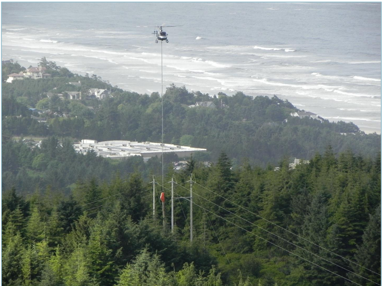
Aerial trimming of Central Lincoln’s transmission right-of-way
