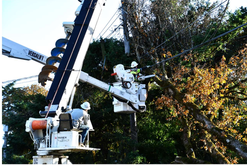
CRPUD linemen restoring power during an outage
