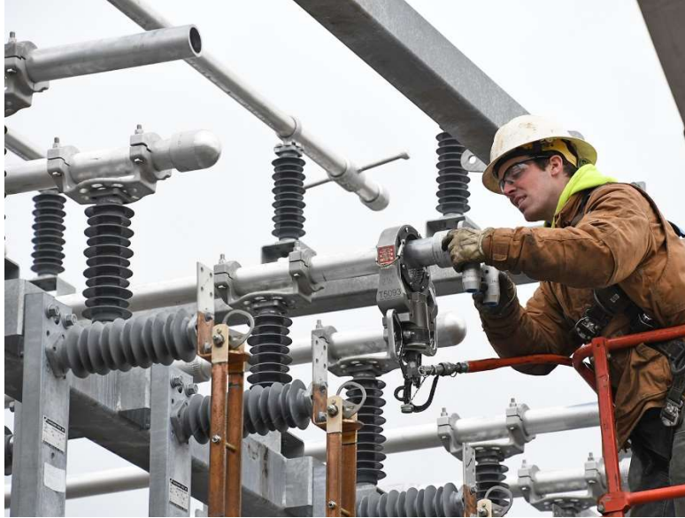
CRPUD lineman performing work on our Betsy Johnson Substation
