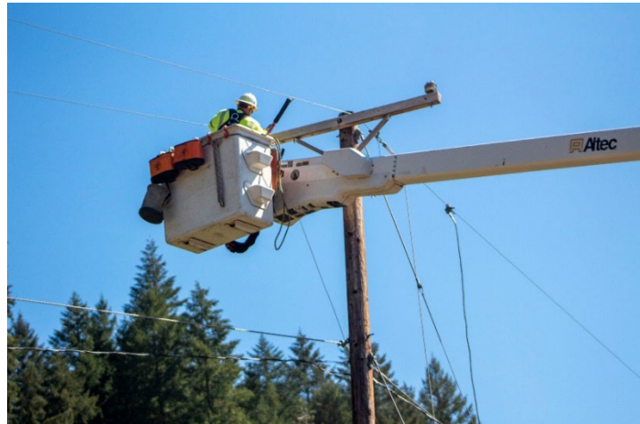
2022 single-phase reconfiguration work
