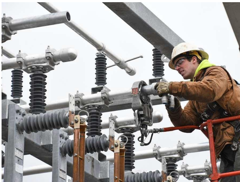
CRPUD lineman performing work on our Betsy Johnson Substation
