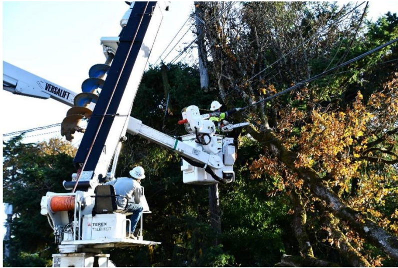
CRPUD linemen restoring power during an outage
