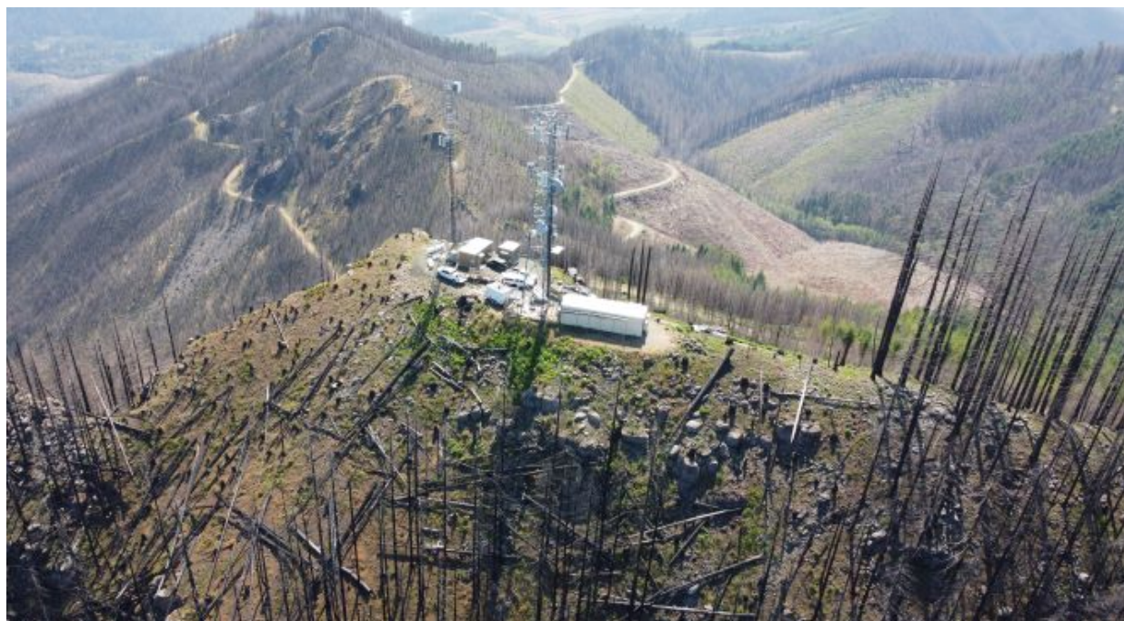
Mt. Hagen Communications Facilities Post-Holiday Farm Fire
