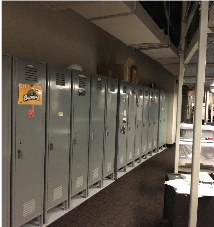
Unbraced Lockers at Level 5
