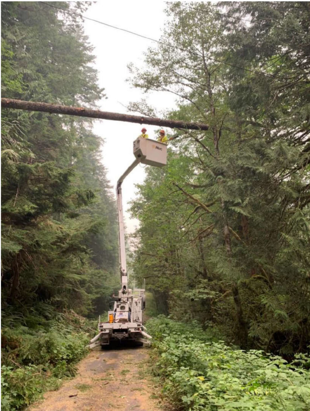
FIGURE 7: FORESTRY BUCKET AND TREE-TRIMMING CREW ON AWRR DEPLOYMENT
