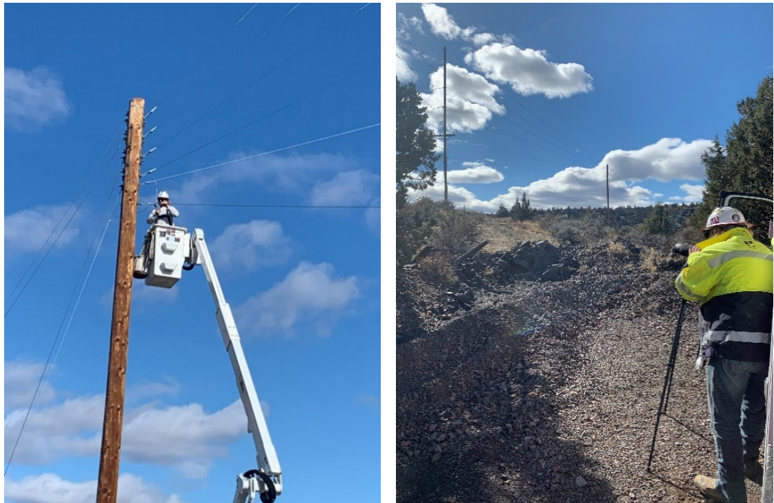
FIGURE 9: PGE INSPECT-CORRECT CREW REPAIRS AND INSPECTIONS USING HIGH-POWER SPOTTING SCOPE
