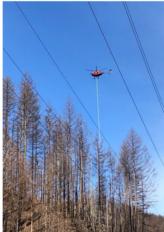
FIGURE 10: HELICOPTER VEGETATION MANAGEMENT
