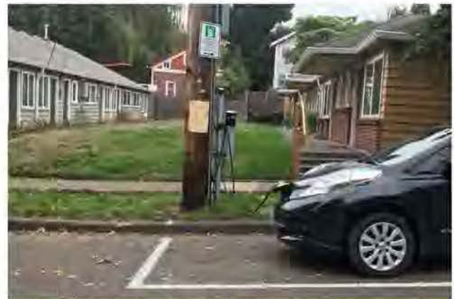
Figure 2. charger on SE 29 th Ave.
