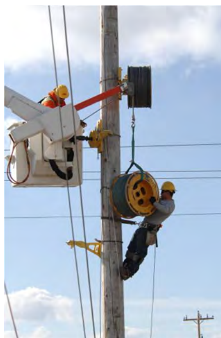
Idaho Power linemen install upgrades.
