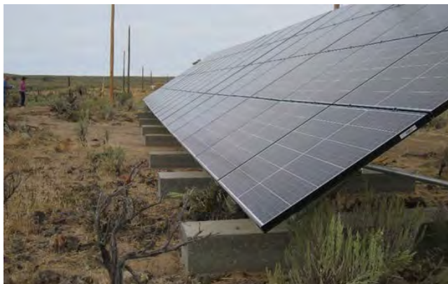
Solar installation as part of the Solar End-of-Feeder Project.
