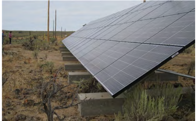
Solar installation as part of the Solar End-of-Feeder Project.
