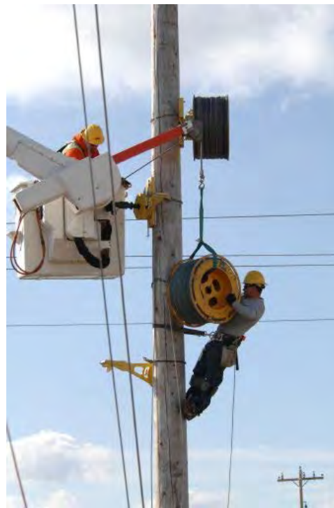
Idaho Power linemen install upgrades.
