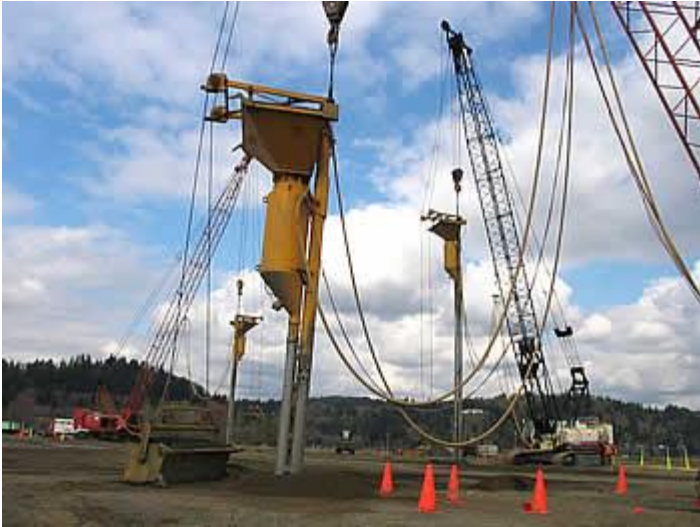
Stone Column Installation
