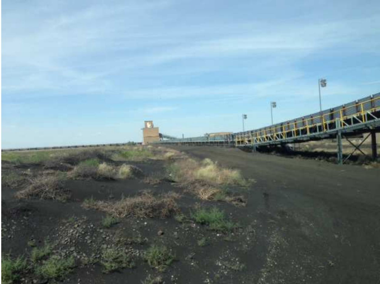
East end of the coal yard, looking at TP-2 from the south
