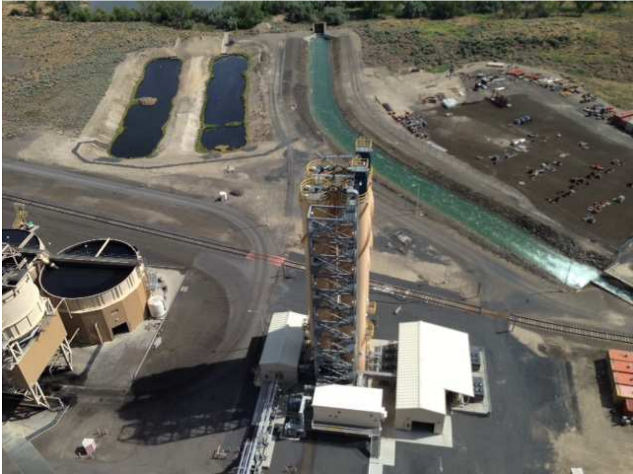
Ash farm, settling ponds, Trona silos & DSI injection system bldgs., circulation water discharge channel
