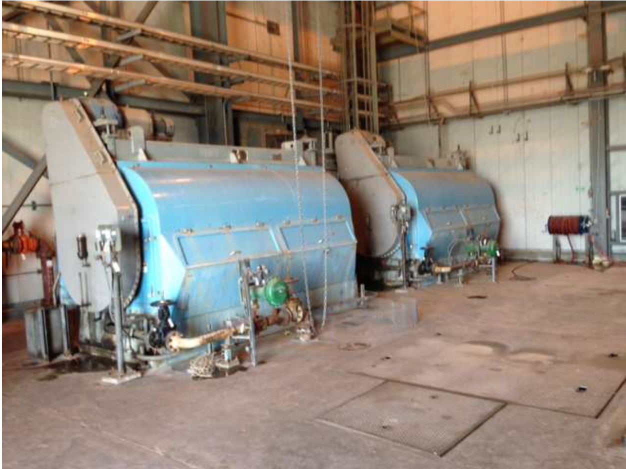
A&B Circulation water travelling screens inside the intake structure bldg.
