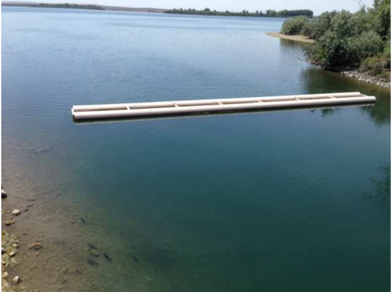
Log Boom made of steel pipe (wave breaker)
