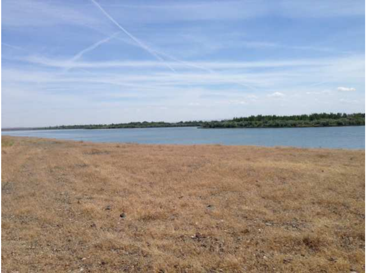
South half of the reservoir from the west end of the divider dike
