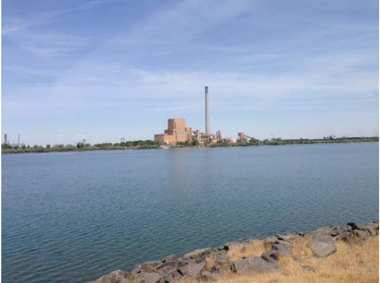
BCP from west end of the divider dike (630 Mw clear stack)
