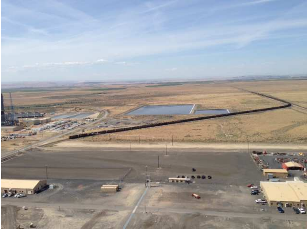
From the roof looking north, lined evaporation ponds, gas plant construction
