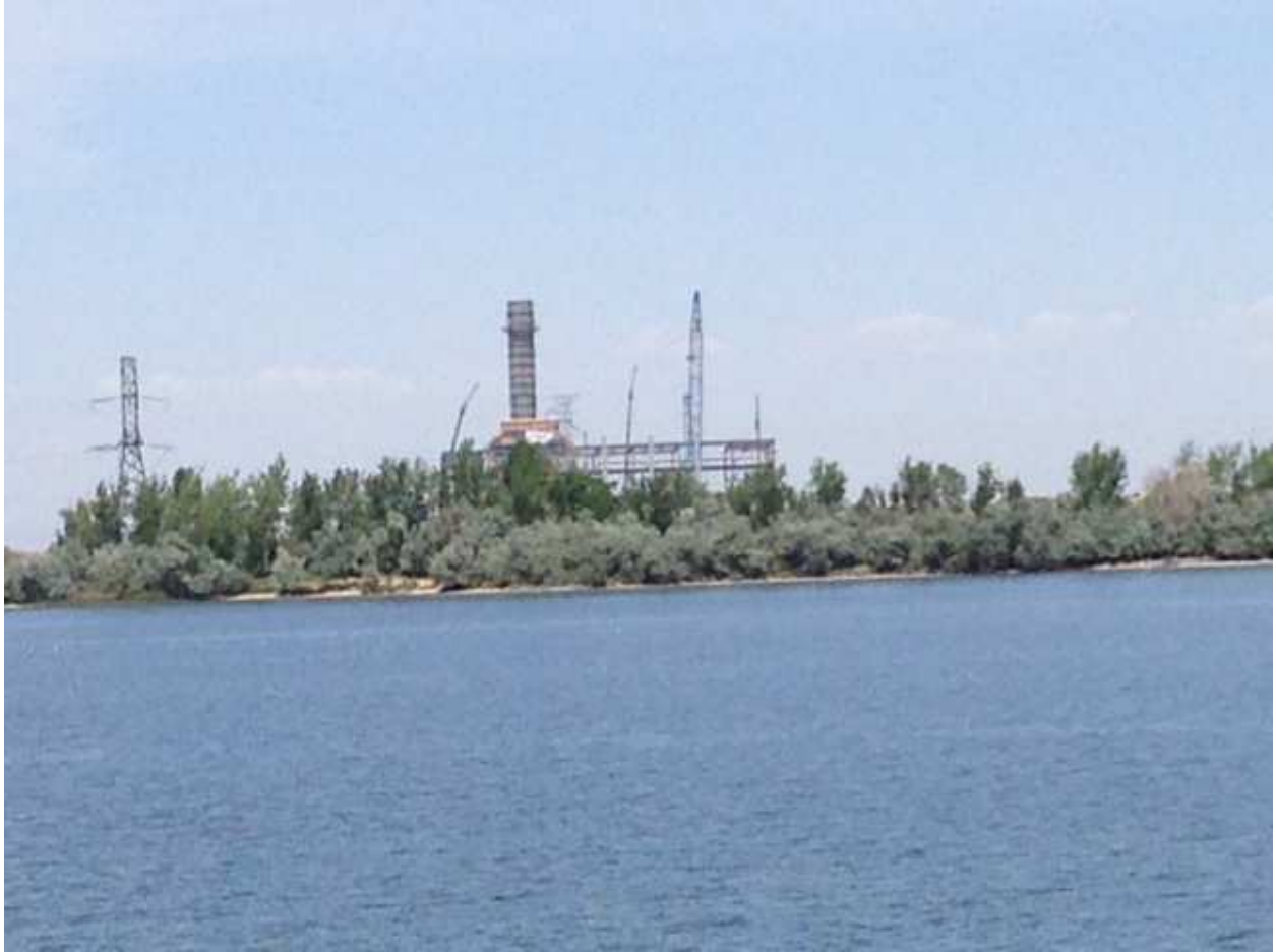
Carty gas plant construction beyond the north shore of the reservoir
