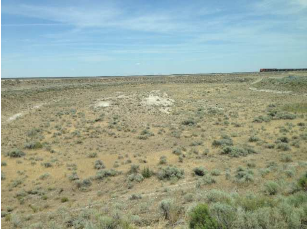
10 Acre, dry, tertiary sewage seepage lagoon
