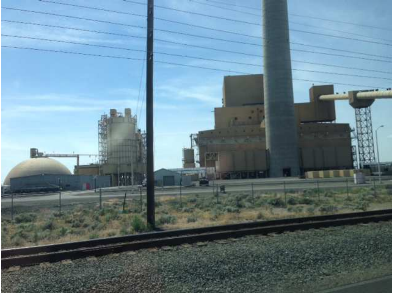
East view of BCP from the coal yard rail loop
