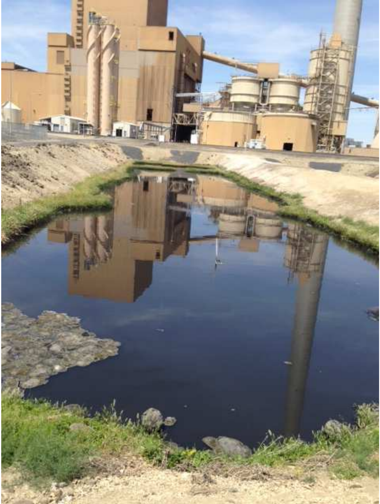
West settling pond looking north
