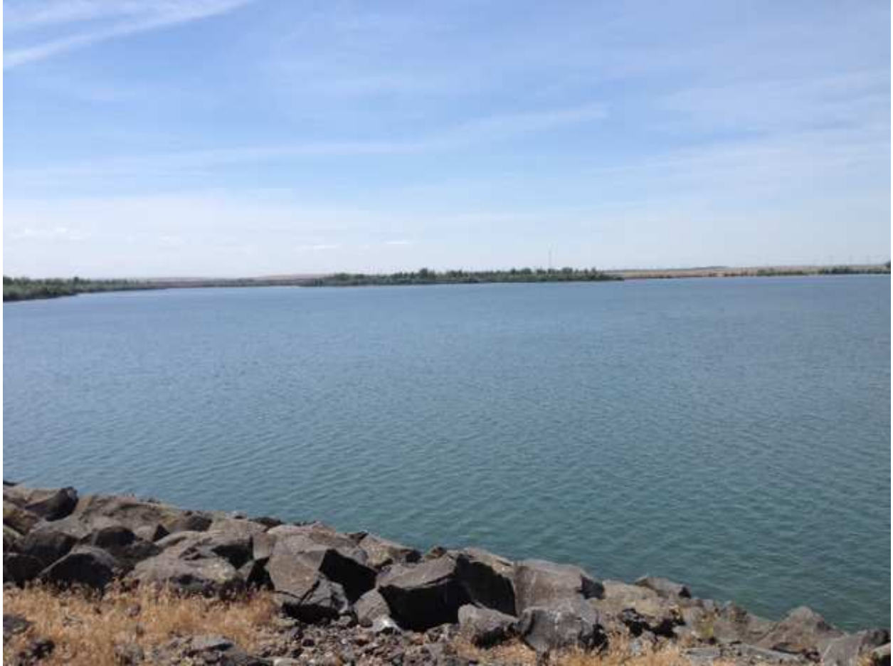
Looking west from the west end of the divider dike
