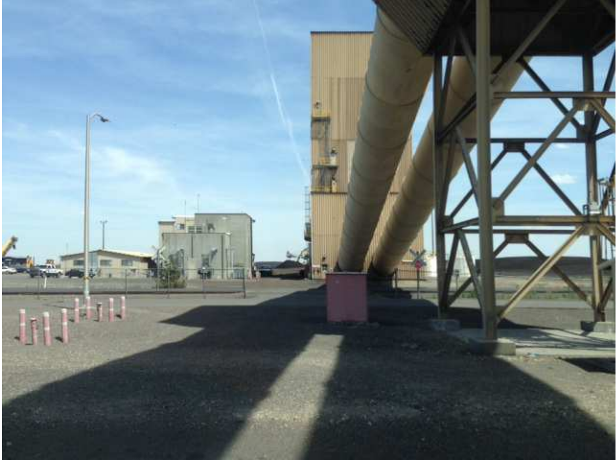
Coal Yard Control Room and shower facilities (left behind pole)
