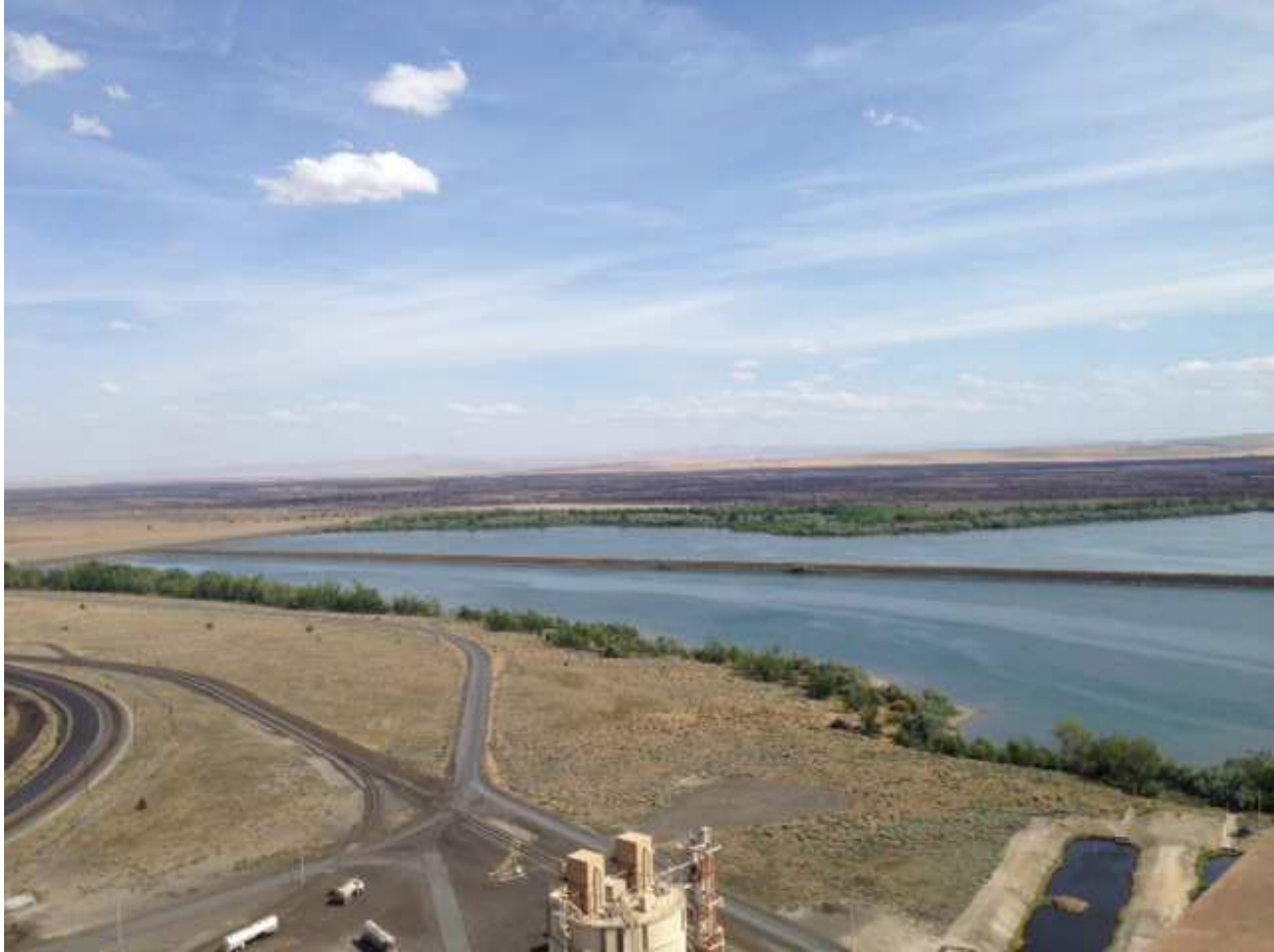
Eastern half of the reservoir, divider dike in the center, ash disposal pit (far away), one settling pond, top of the fly ash silo (two bag houses on top)
