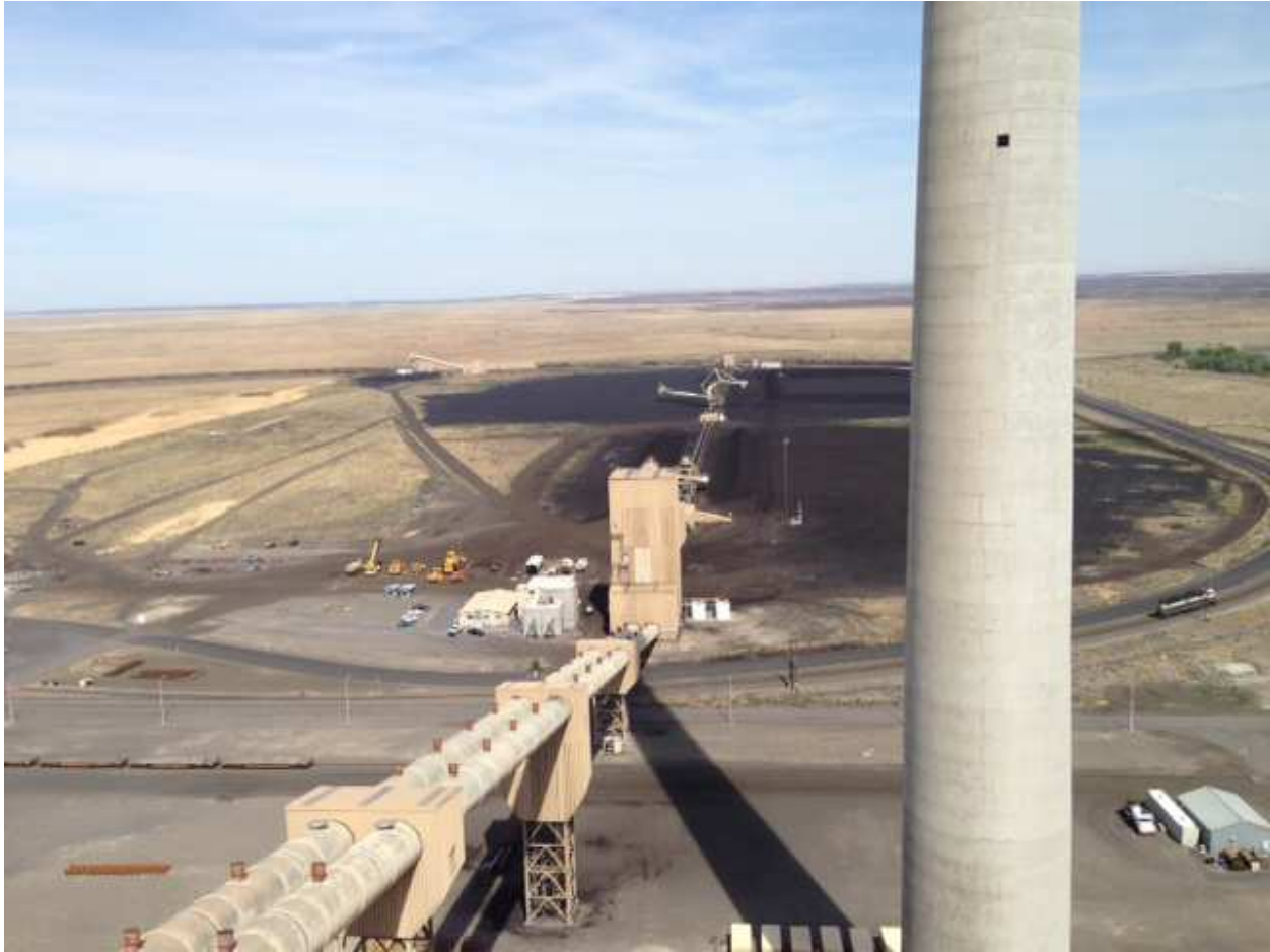
From the roof looking east at the coal yard, lube oil shack in lower right corner
