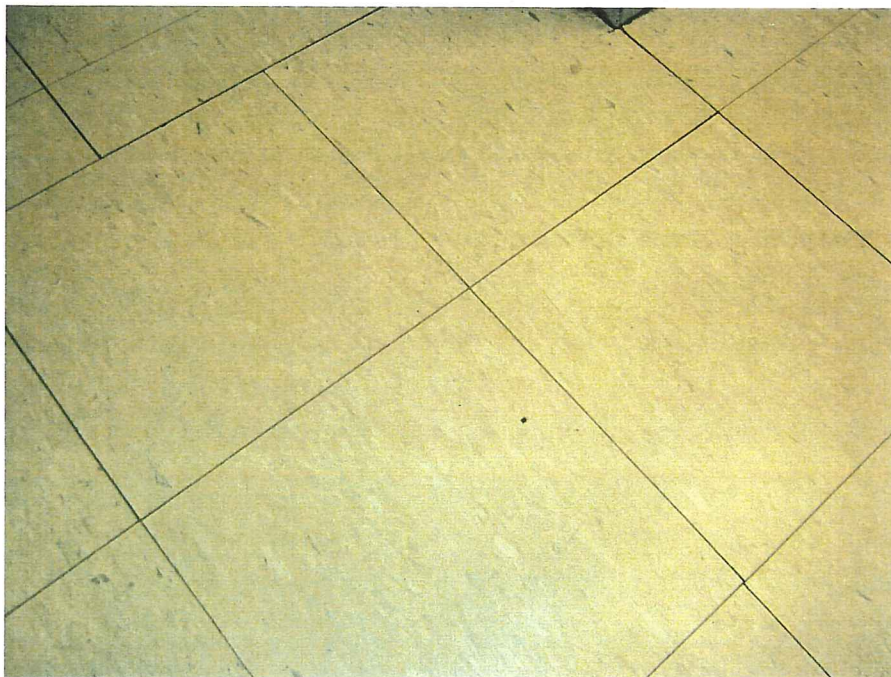
BOARD-66 Floor Tile, 12" x 12" Beige Streaked and Black Mastic
