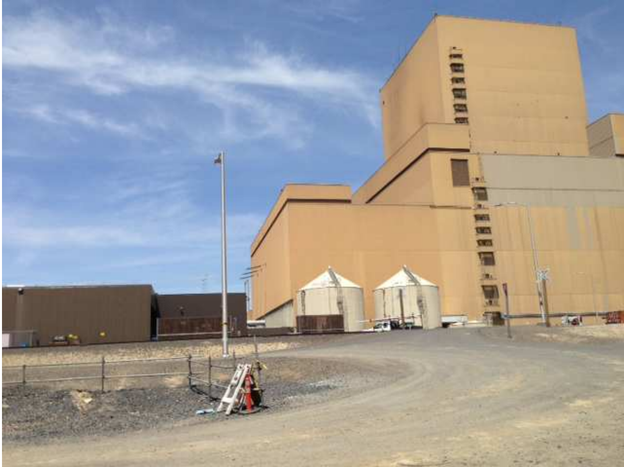
View from the intake structure looking NNE, l <-> r, warehouse, condensate storage tank, demineralized storage tank
