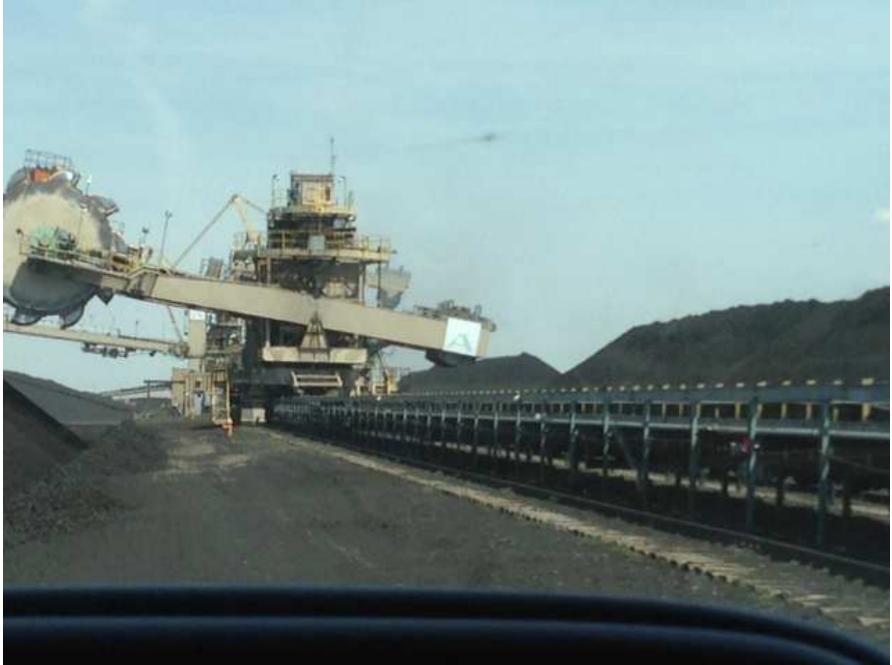
Stacker/Reclaimer #3 looking from the west
