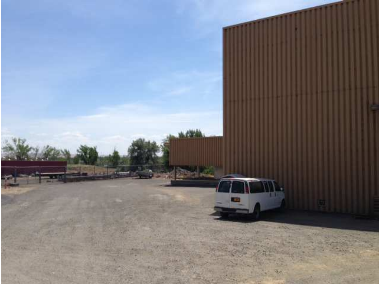
Intake structure bldg.
