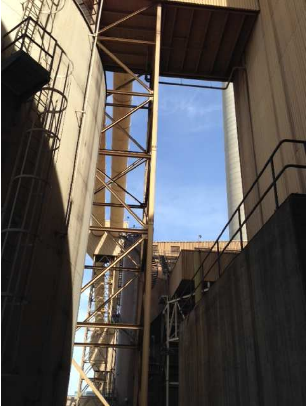
Filtered water storage tank (left), PAC silo (center), Neutralization sump (right).
