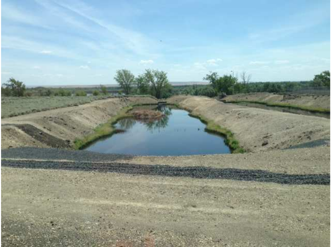
West Settling Pond
