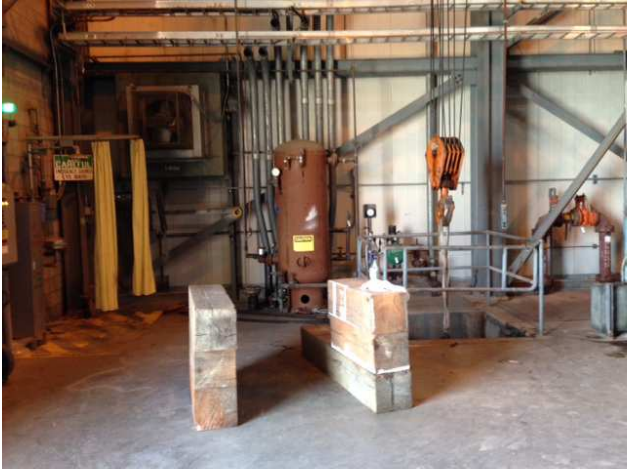
Intake bldg. air receiver and trash basket pit for travelling screens. Cribbing in the foreground.
