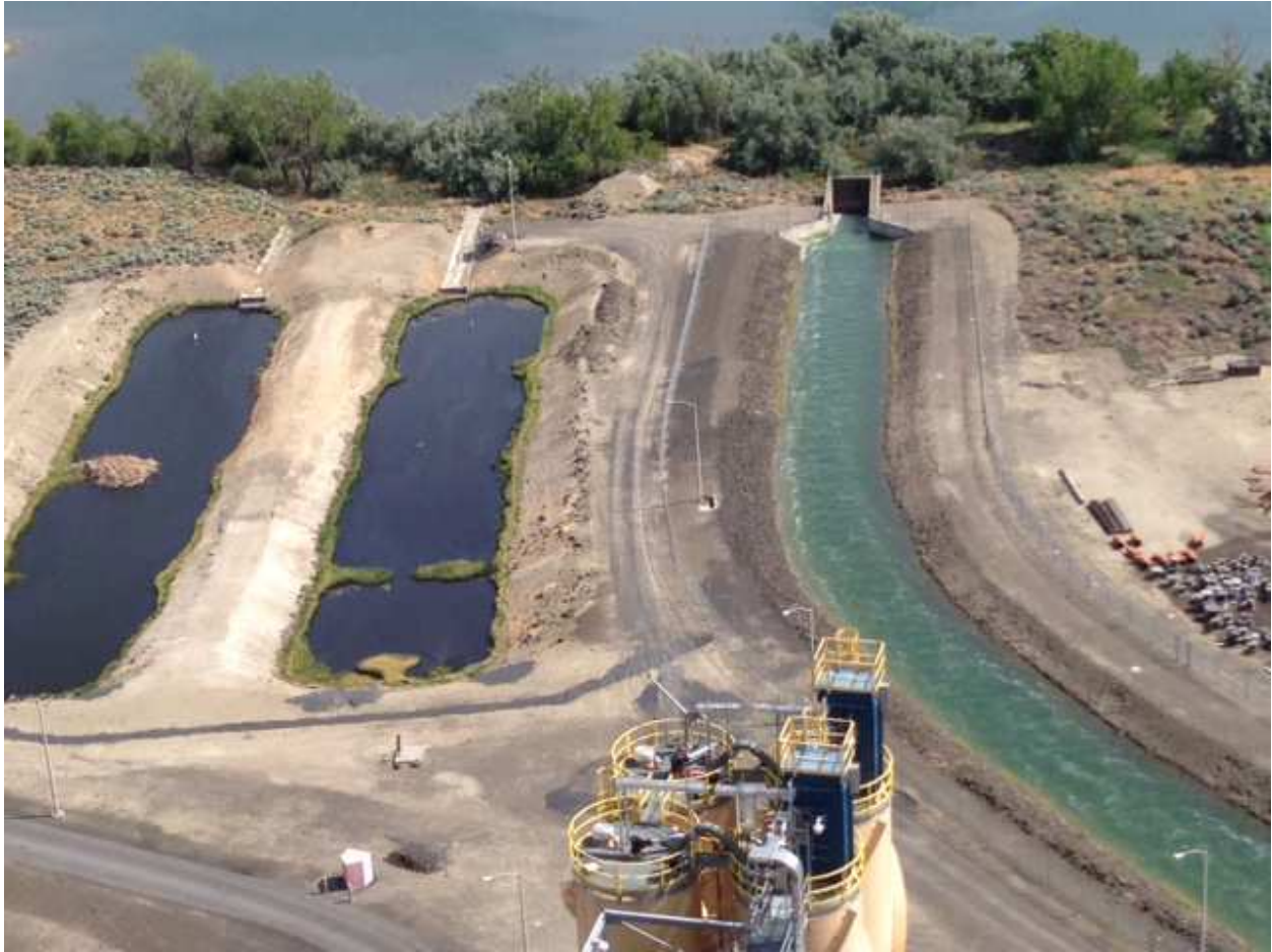
Trona silo baghouses, settling ponds, discharge channel
