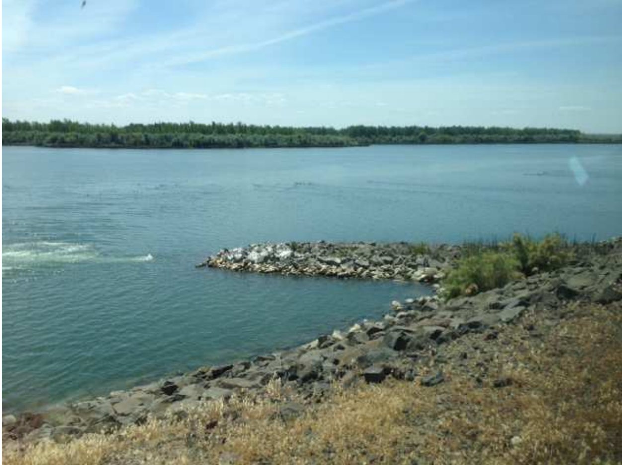
Circulation Water Discharge on south side of the divider dike
