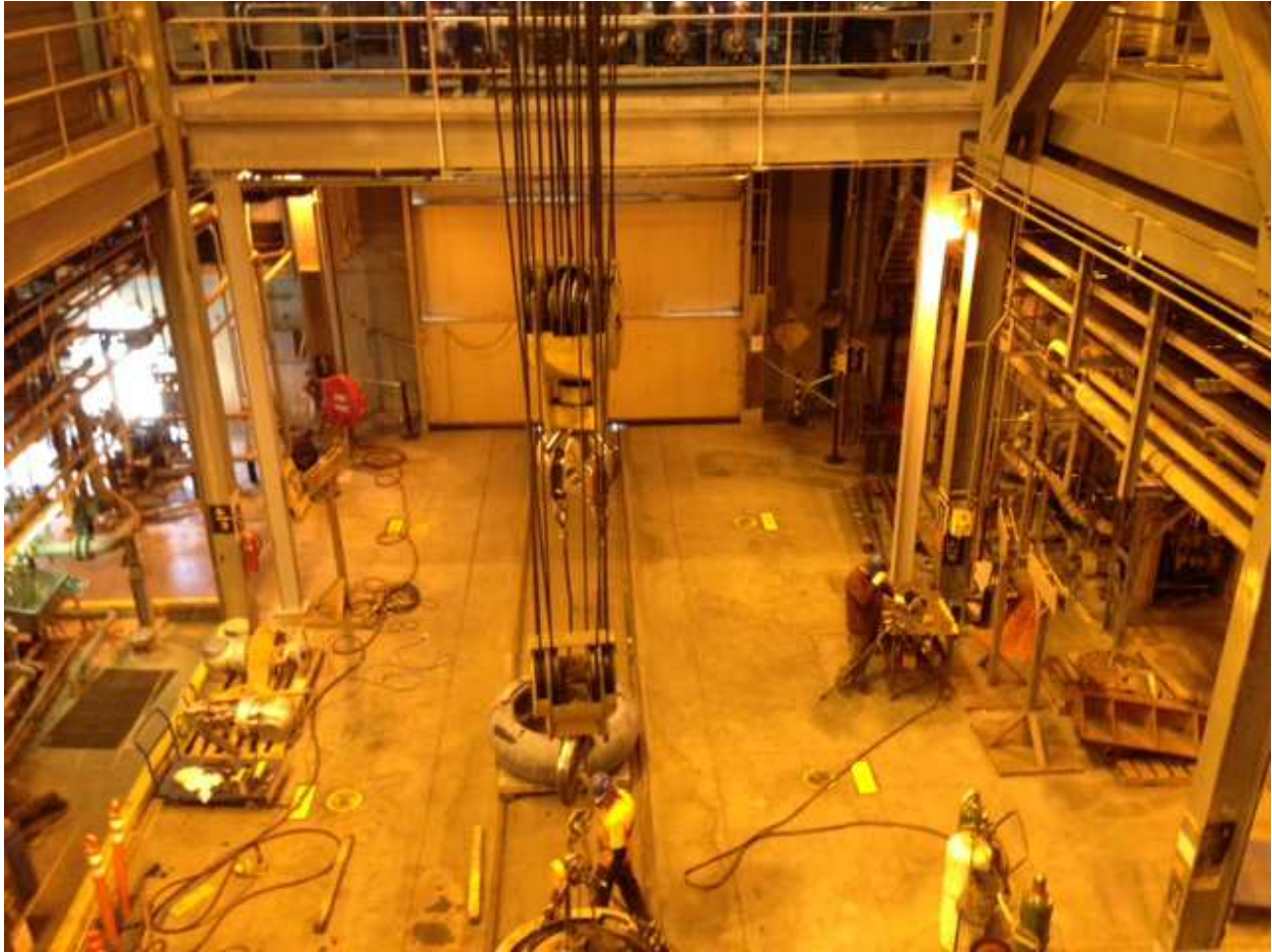
Crane bay, rigging a pulverizer wheel
