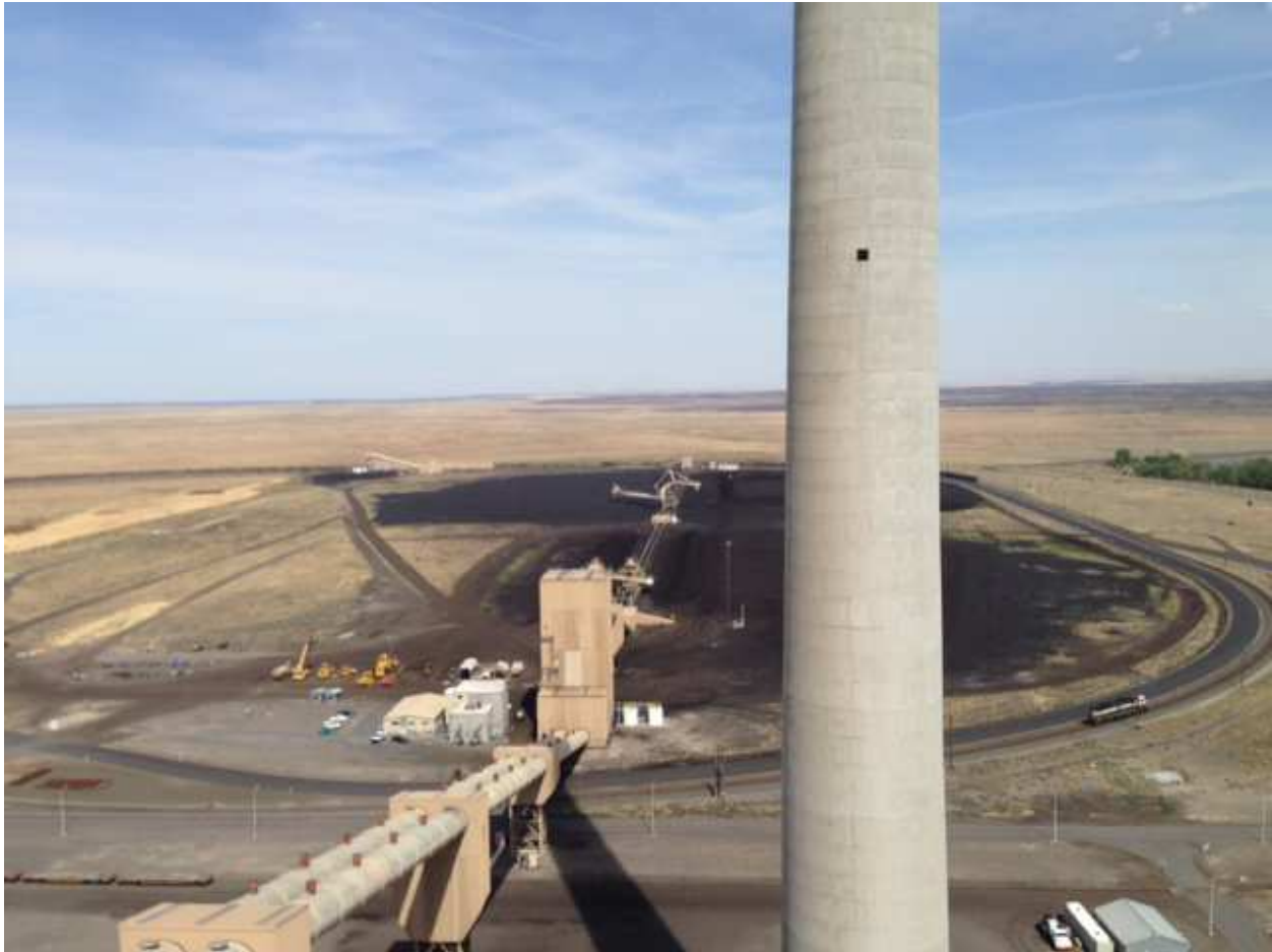
Chimney, coal yard rail loop, stacker/reclaimers (2), crusher bldg., long tubes (coal belt protection)
