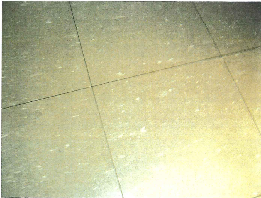
BOARD-113 Floor Tile, 12" x 12" Brown w/ White Specks and Black Mastic
