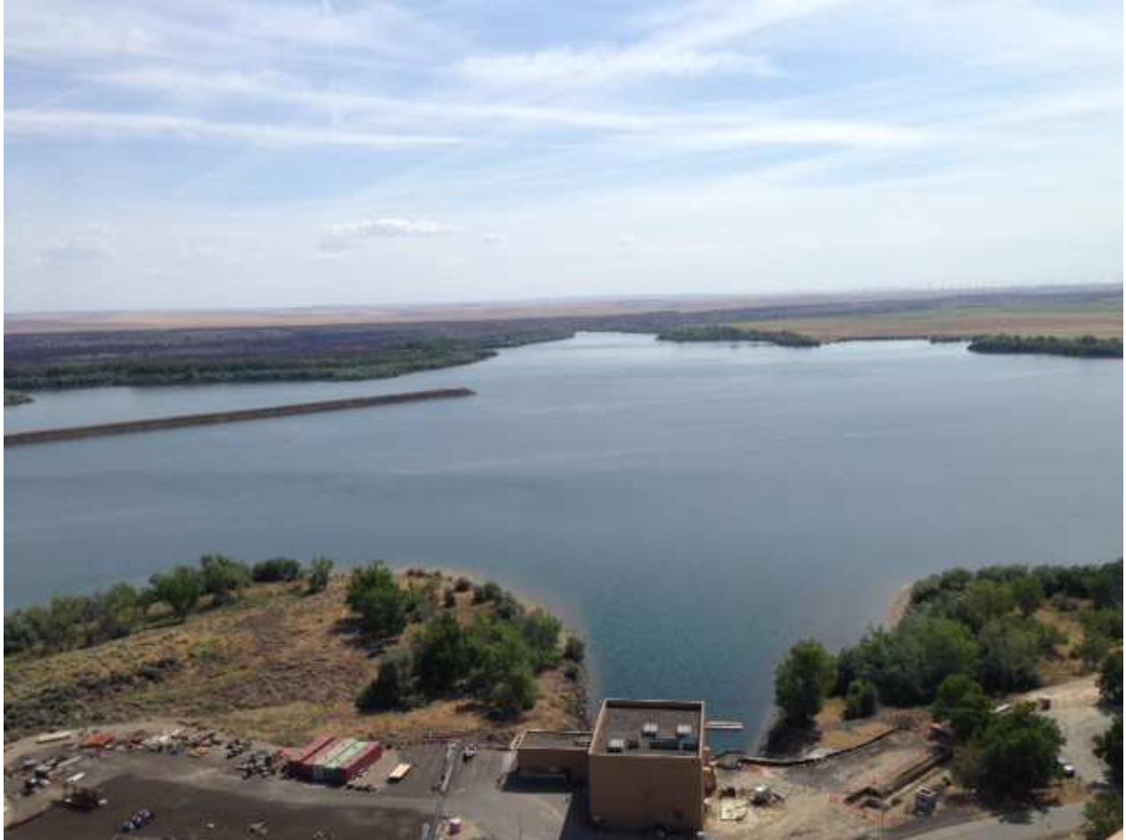
Western end of the reservoir with intake structure in foreground
