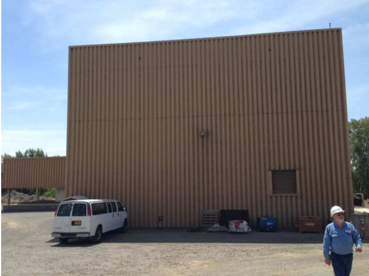
NE wall of the intake structure bldg.
