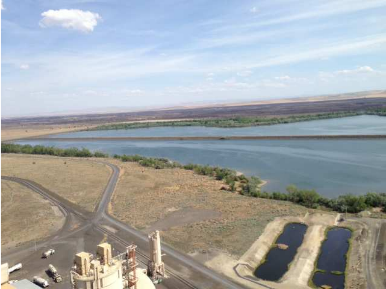
Ash handling facility, fly ash silo, dome, and load out silo, settling ponds, reservoir, ash disposal pit, beautiful eastern Oregon horizon
