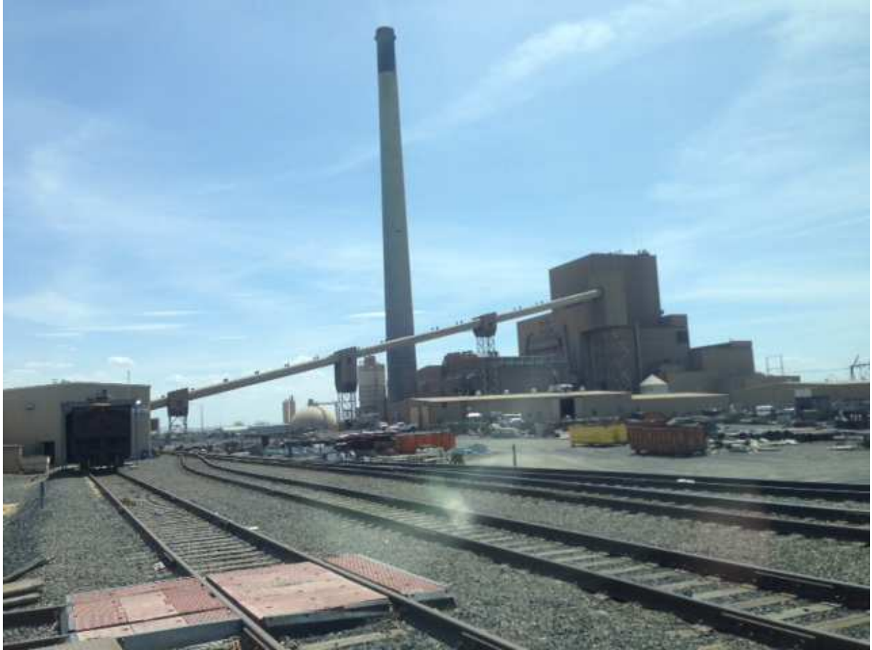
Rail car repair shop viewed from the north
