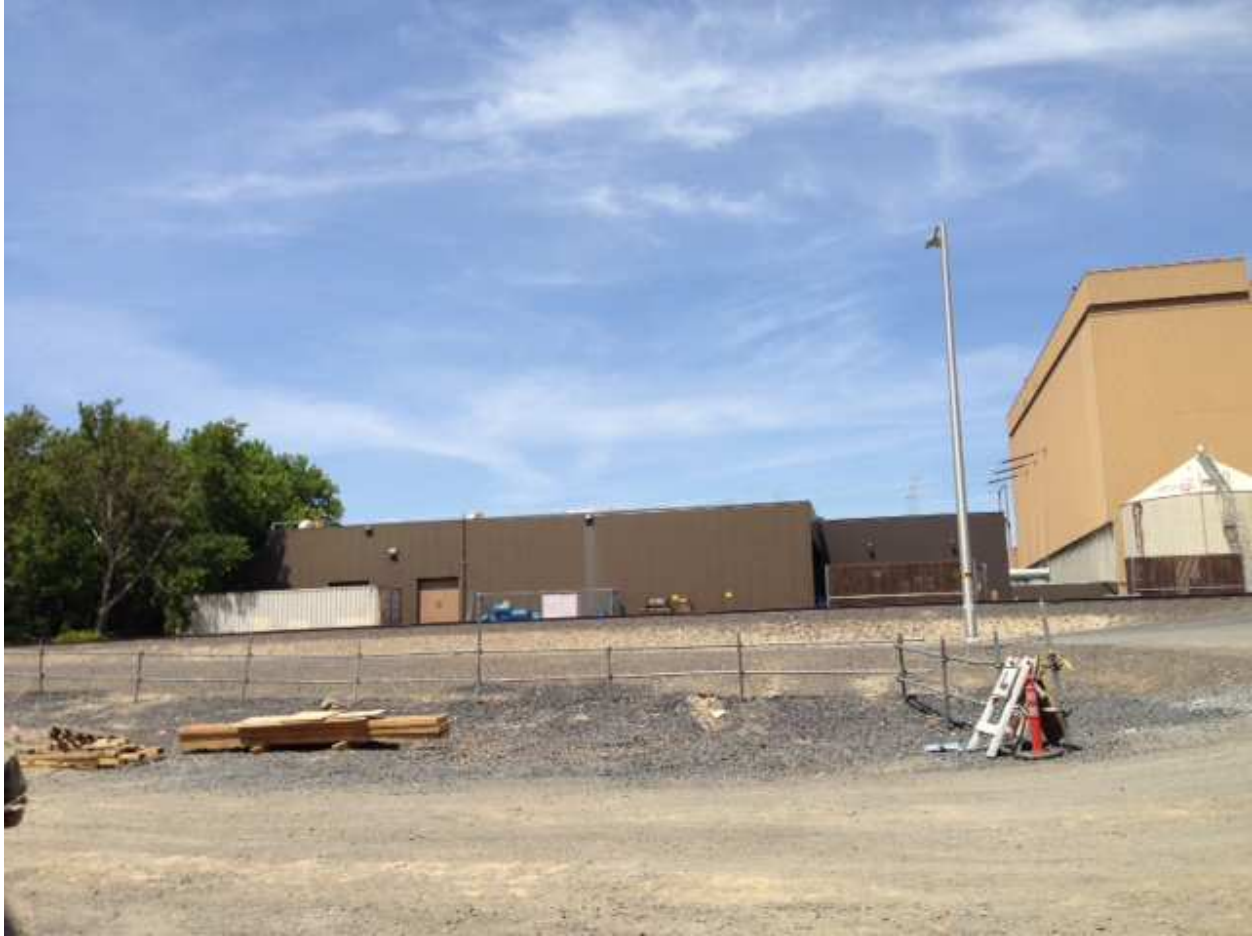
Warehouse end of the admin bldg.
