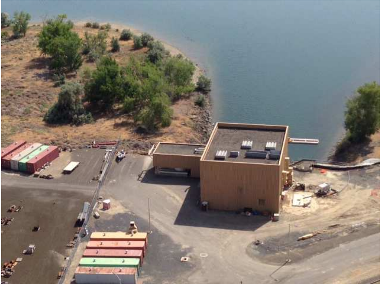
Intake structure and intake channel
