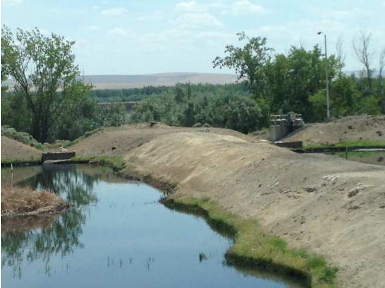
More of the settling ponds- sump pumps are in the pill box to the right
