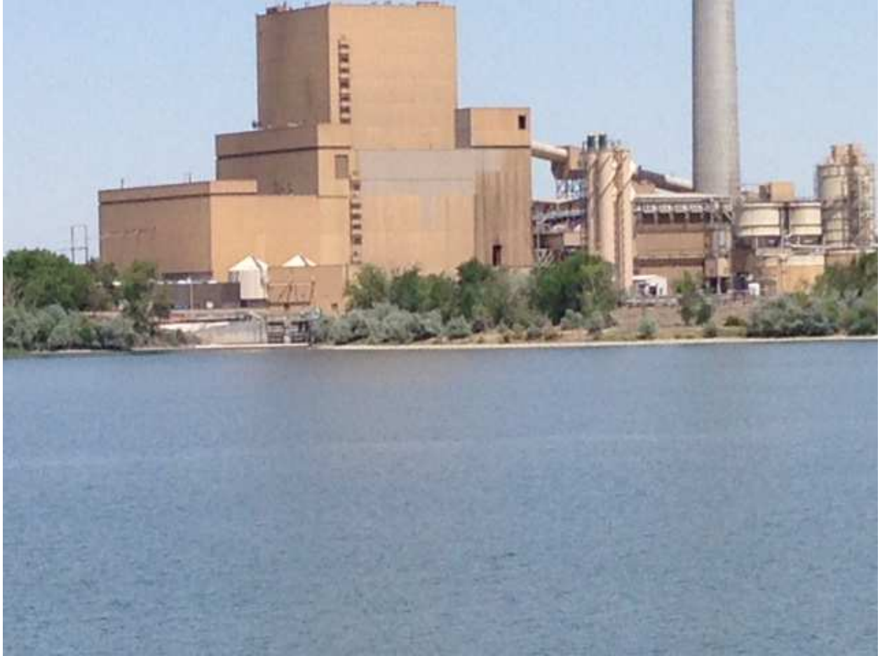
Intake Structure from the divider dike
