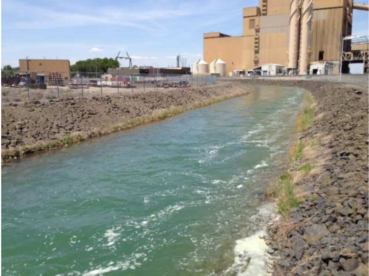
Discharge channel looking upstream
