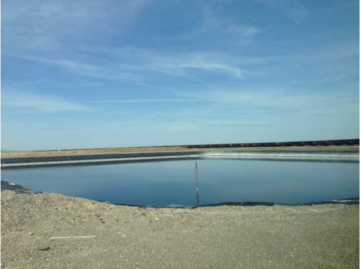
2 Acre lined evaporation pond
