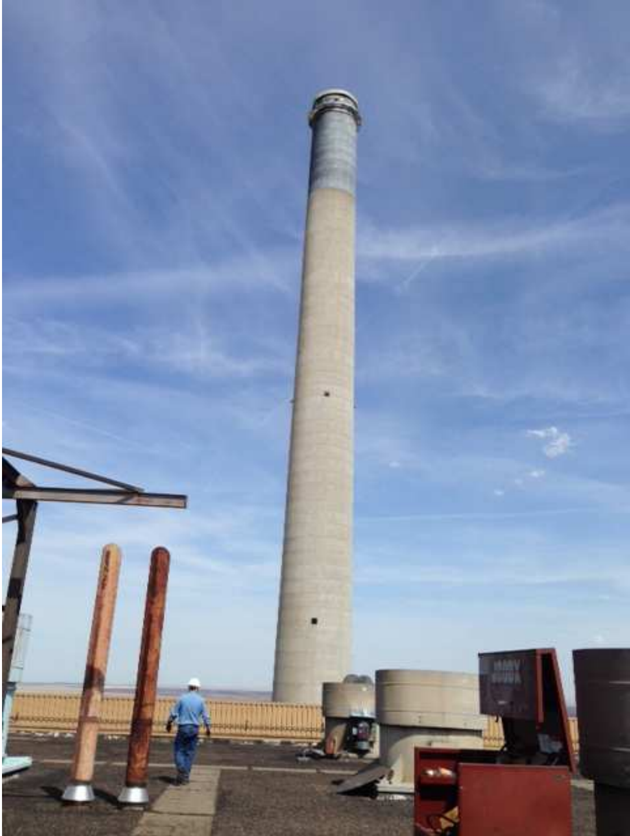
Mass blowdown pipes and the chimney (656 foot tall)
