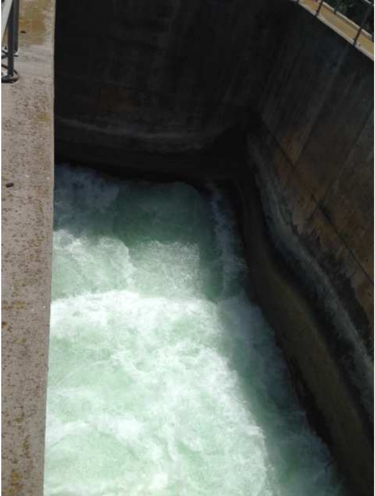
Discharge channel looking down into the outfall structure
