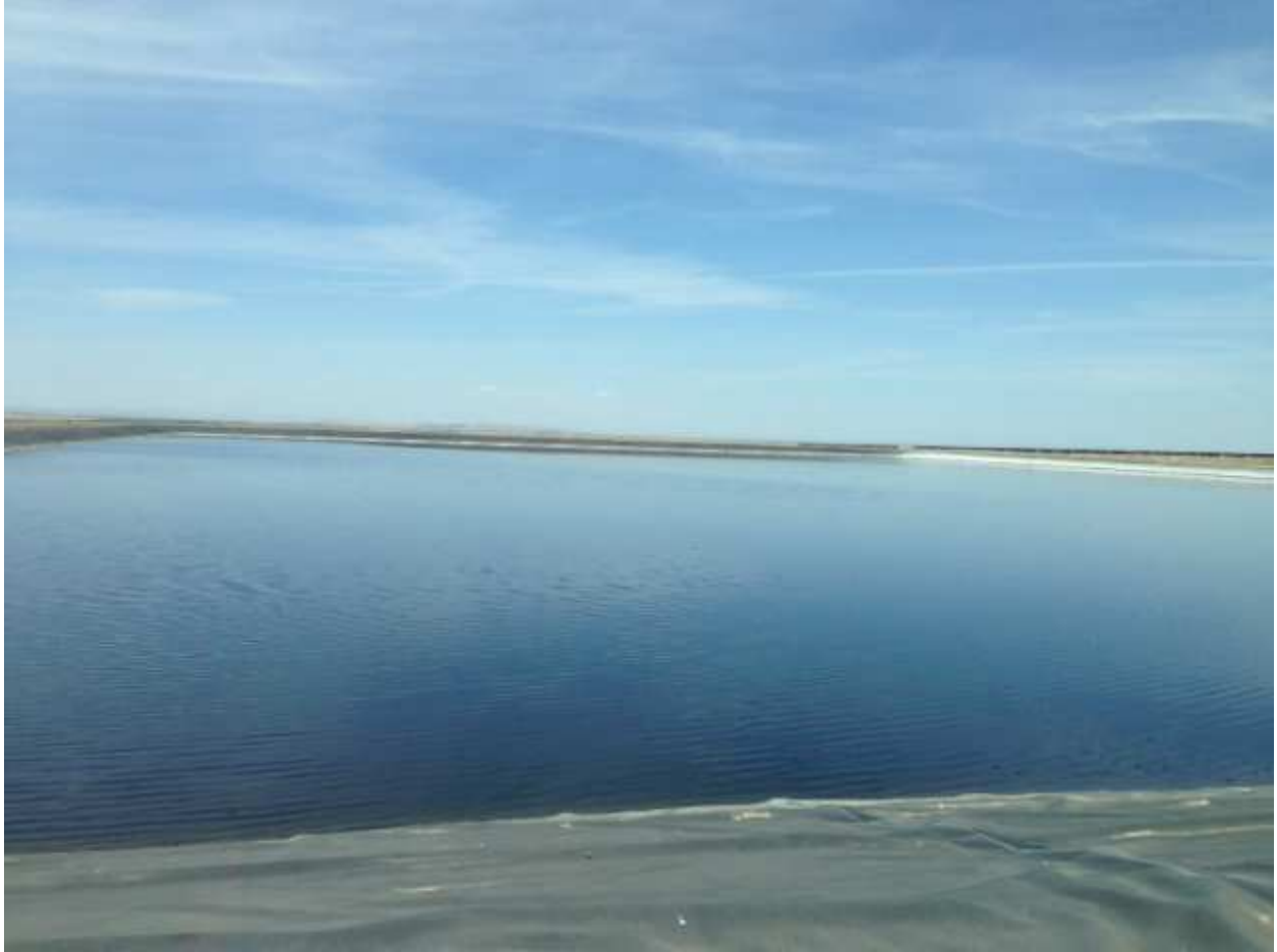
10 Acre lined evaporation pond, north of the plant
