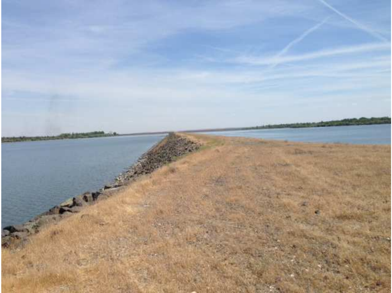
Divider dike from its west end
