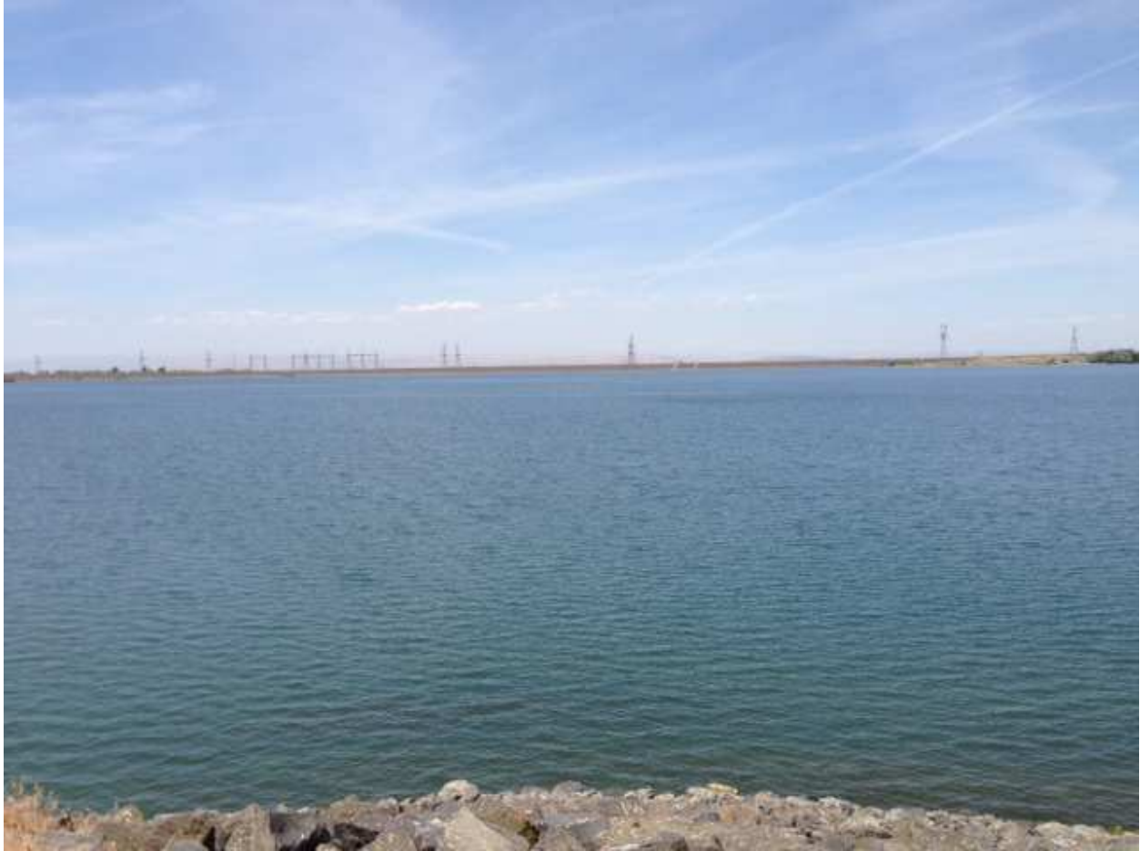
Looking at the West Dam from the west end of the divider dike
