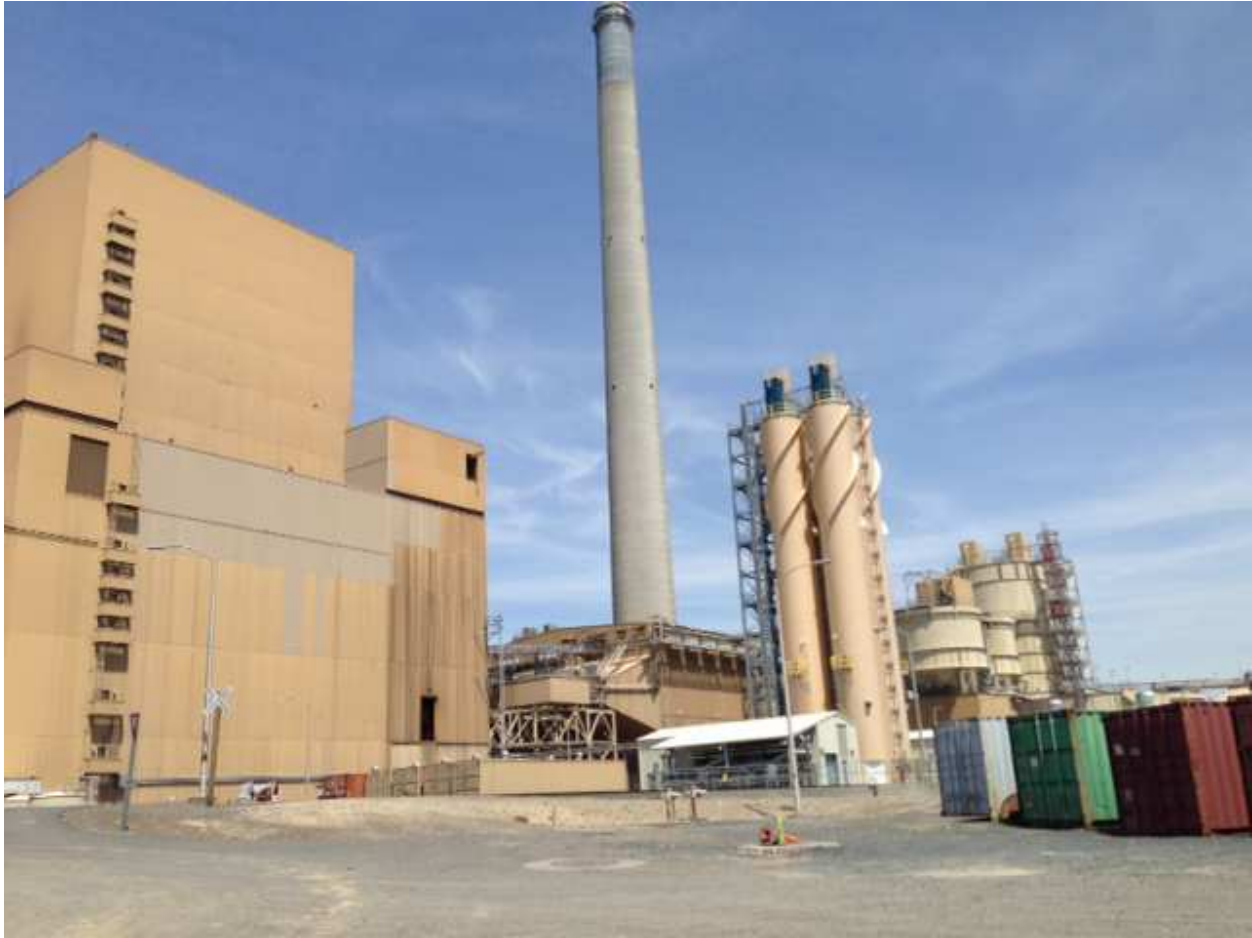
View from the intake structure looking NE
