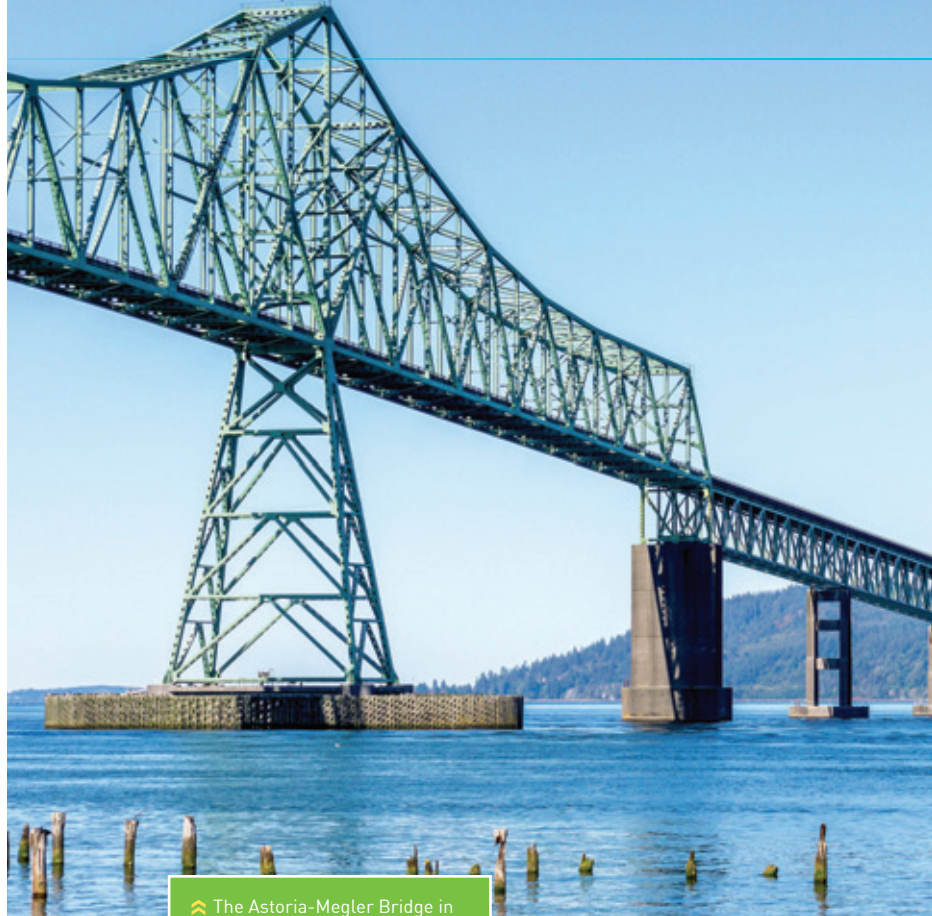
📍 The Astoria-Megler Bridge in NW Natural's service territory.
