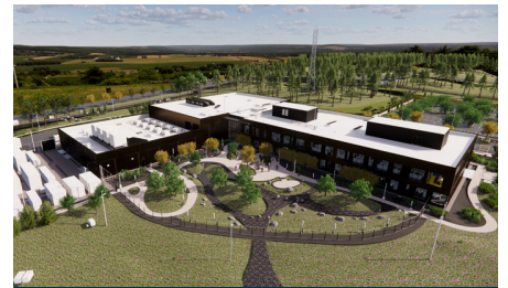
Integrated Operations Center
